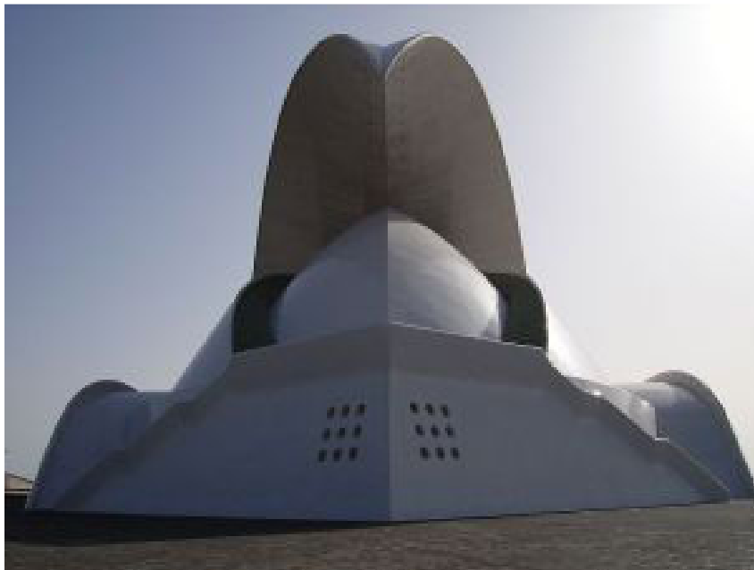
Figure 28 - Finished view of the 50 meters wing over the concert hall
