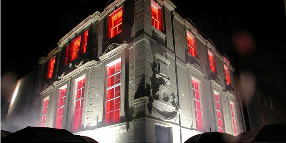
Figure 16 - Egg Theatre in Bath, UK - Example of a theatre with smaller windows that has highlighted itself by an inviting reflection of red light to outside
