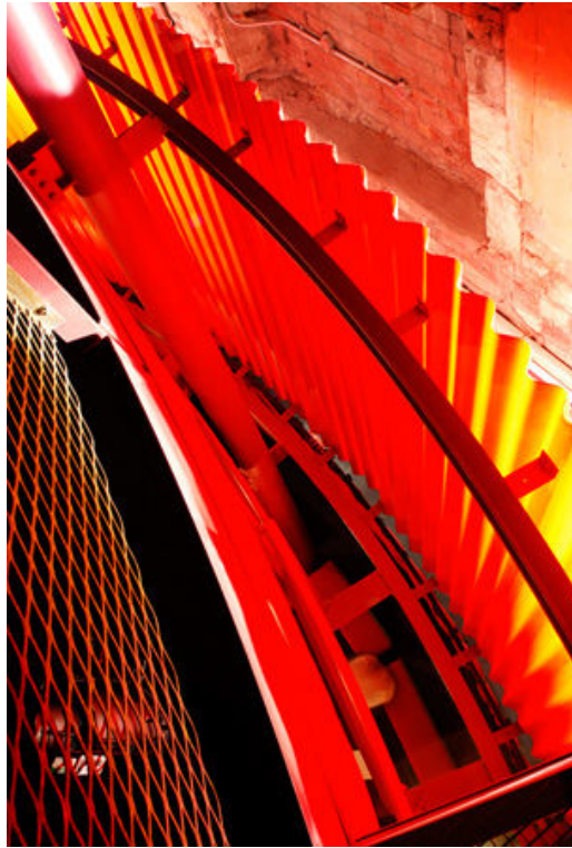
Figure 54 - Corrugated red plastic sheets reflecting the light from outside
