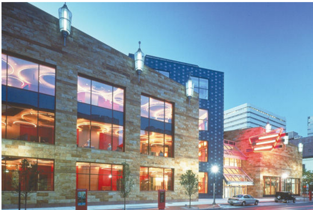
Figure 15 - Whitaker Centre, Pennsylvania, US - Lobbies are unpopulated during performances and when unused, so it is wise to design a second interior lighting feature that highlights the theatre's presence
