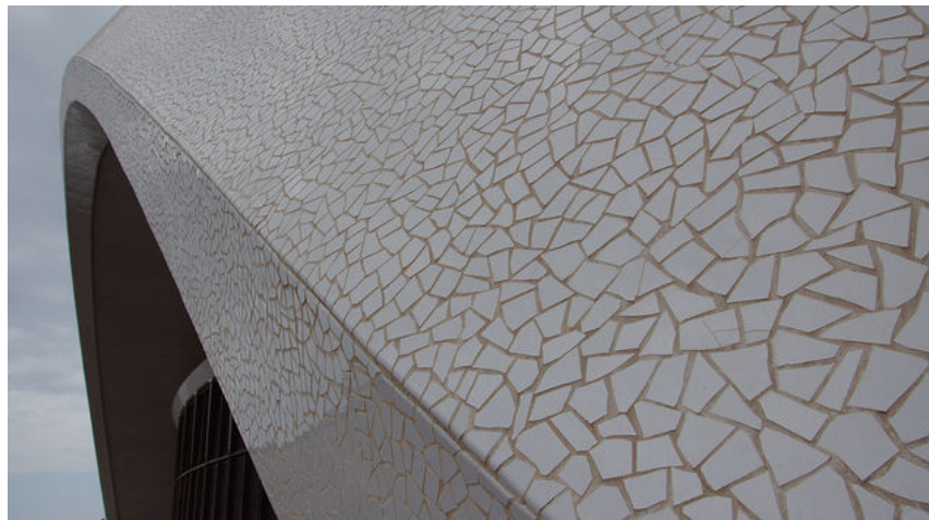
Figure 23 - The glowing facade is created with carefully installed broken ceramic tiles
