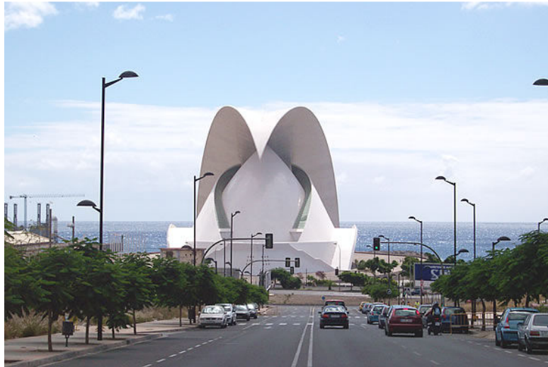
Figure 22 - View of the Auditorium from Calle Fuente De Sta Cruz
