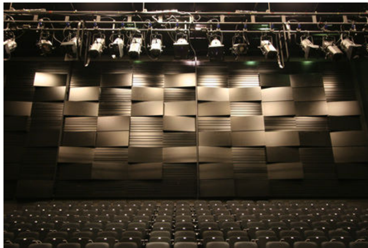
Figure 723 - Rear wall sound reflectors
