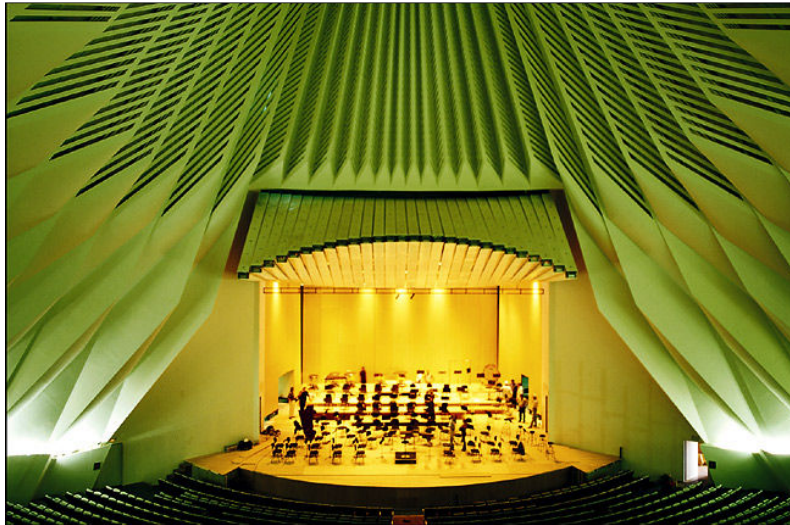
Figure 44 - concertina screen of vertical aluminum slats, which when opened lift up into the auditorium to act as a sound-reflector above the orchestra pit
