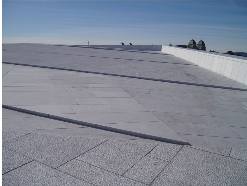
Figure 63 - The Carpet or the Opera House's Roof Made with Italian La Facciata Marble
