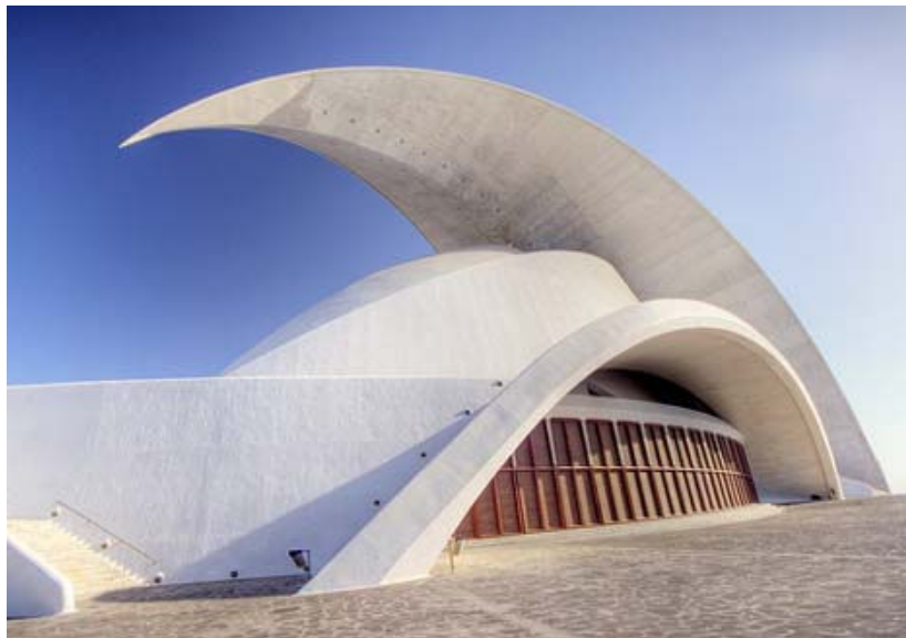
Figure 26 - Concrete arches with glass entrances, spanning 50 meters, transfer the loads to the foundations
