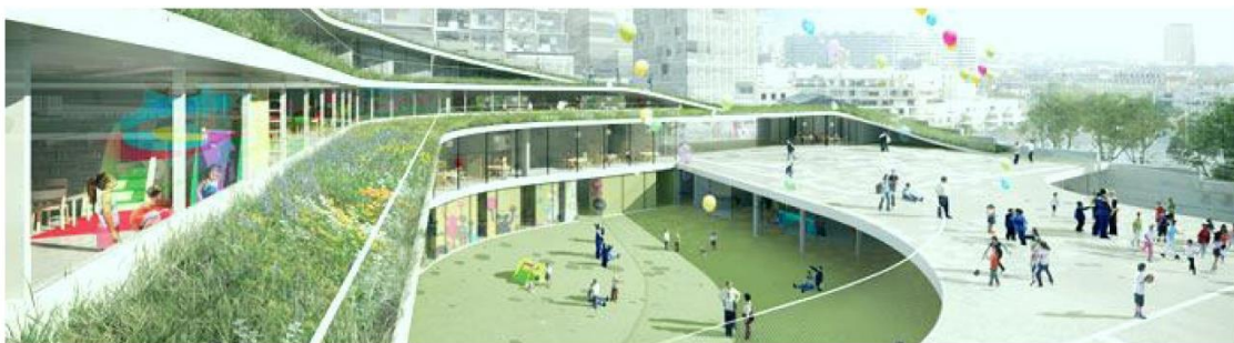
Fig. 4.19 – Brillant primary school, C&D Architects
