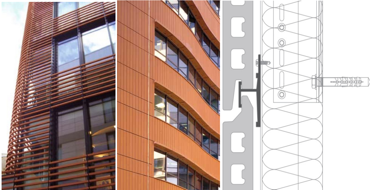
Figure 4-32: Terracotta Façade Installation
