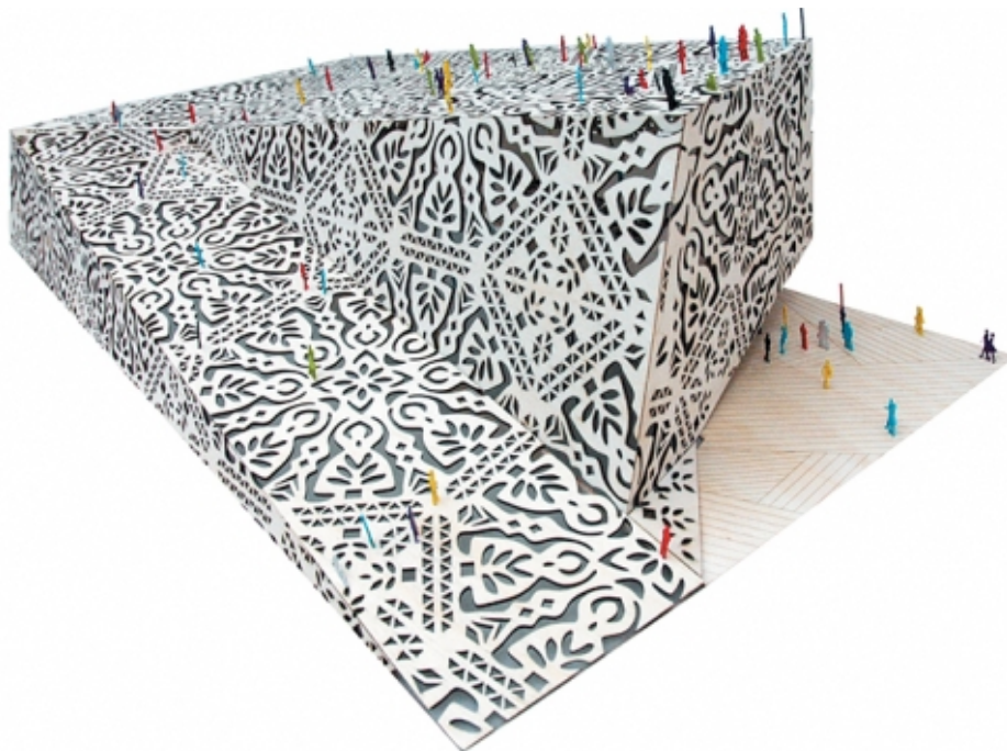
Figure 1-12: Polish Pavilion in Shanghai EXPO 2010
