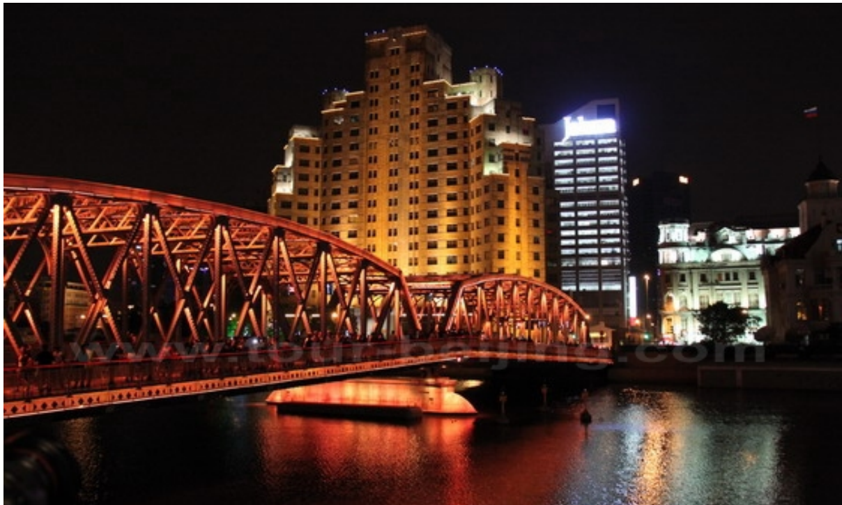
Figure 4-16: Waibaidu Bridge Over the Suzhou Creek
