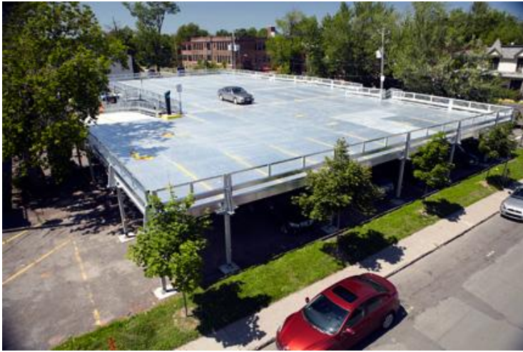
Fig. 3.20: a foundationless single story parking
