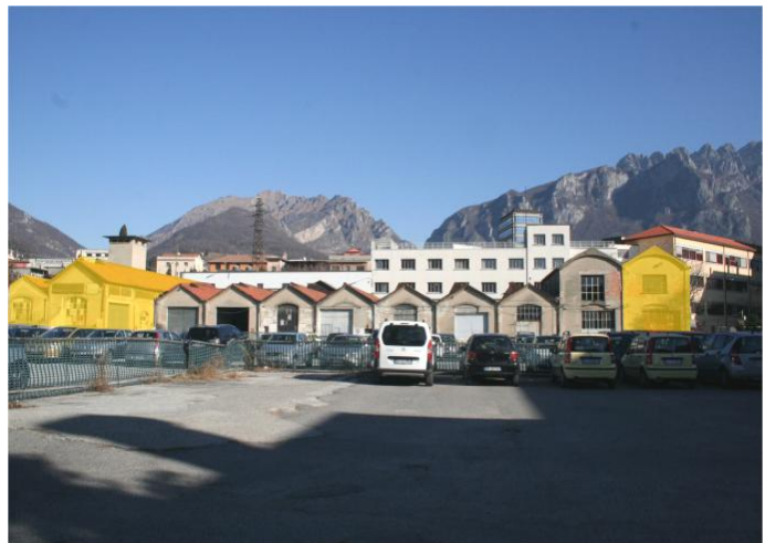
Fig. 3.4: the demolished parts are painted by yellow
