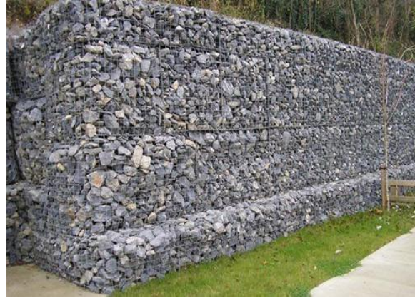
Fig. 3.23: typical gabion wall
