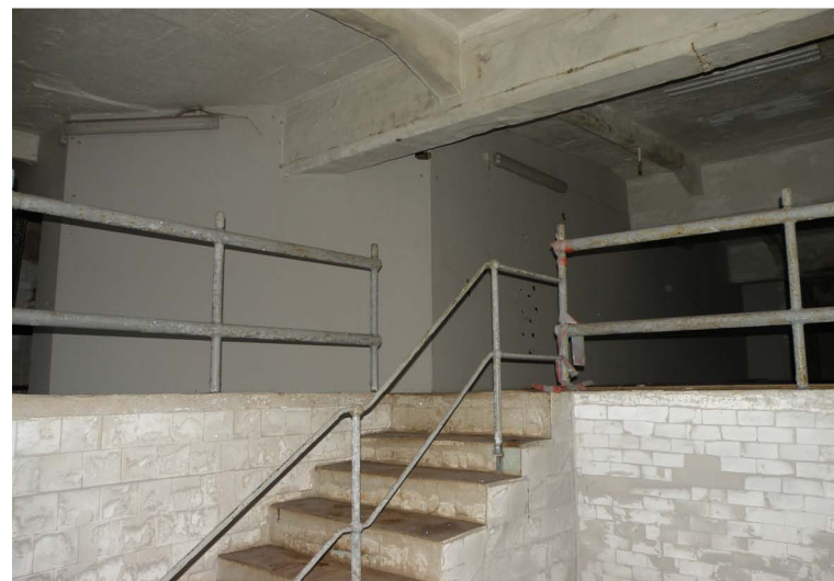
Multifunctional's space upper area
