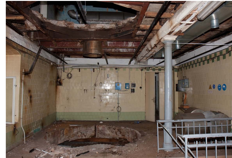
1st floor space
