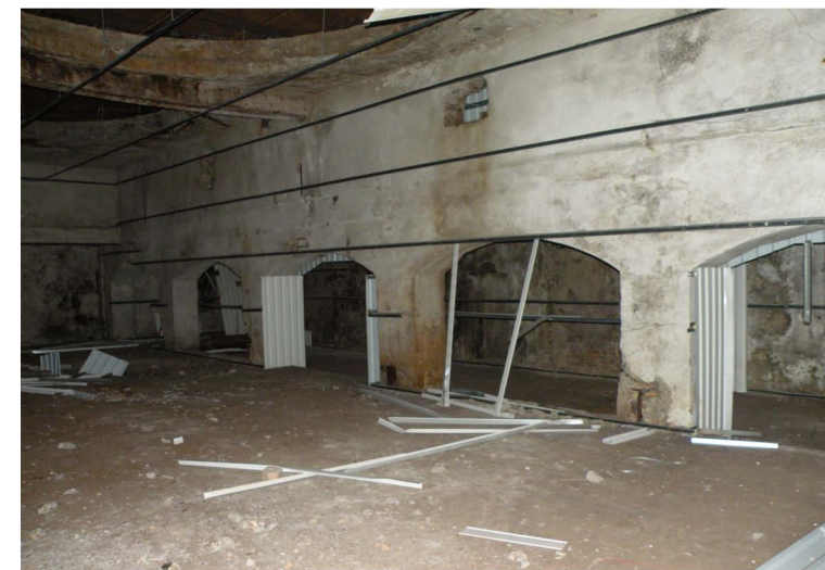
Multifunctional space's lower floor
