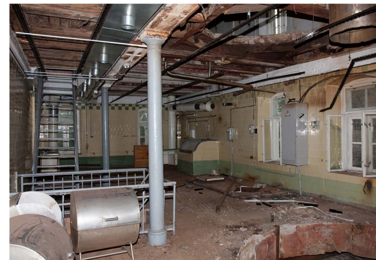
1st floor space
