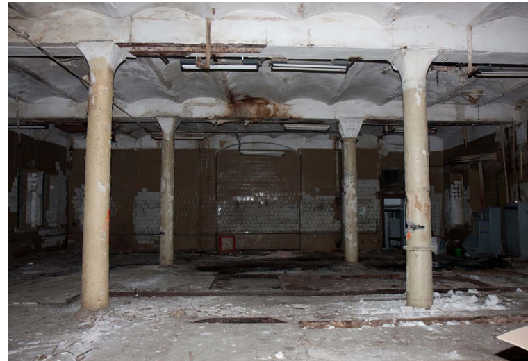
1st floor space
