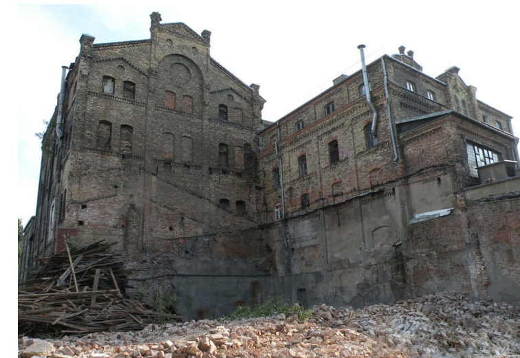
Dismalted South-West area
