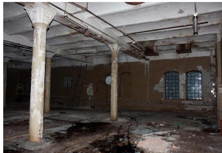
1st floor space
