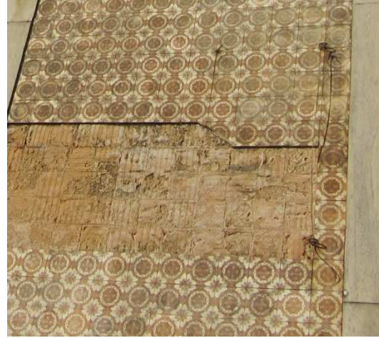
Figure 4.4 - Degradation level 4
