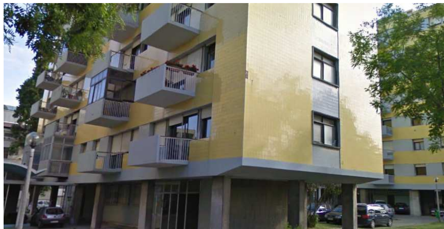
Figure 3.14 - Block of flats in Avenida do Brasil
