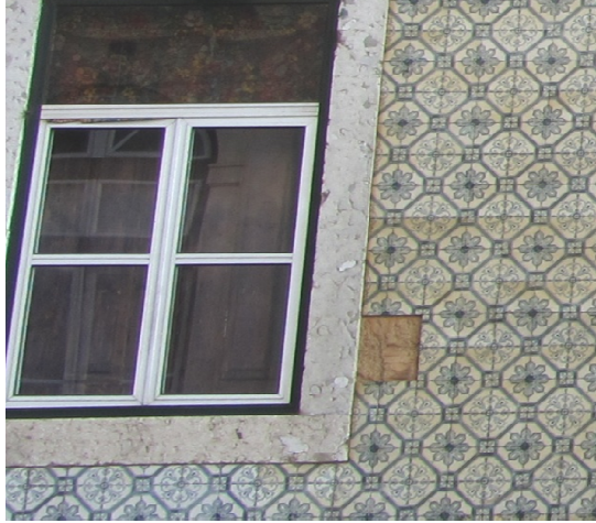
Figure 4.3 - Degradation level 3
