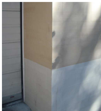
Figure 3.10 - Façade recently renovated
