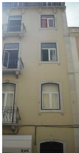
Figure 3.12 - Façade recently renovated
