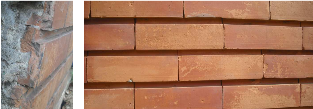
Figure 3.15 - Bricks façade of the Encarnação Norte market
