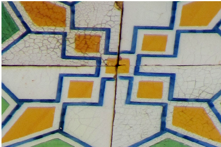
Glazing cracking
