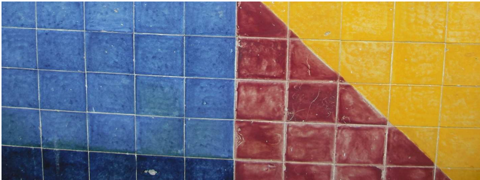
Figure 3.16 - Portion of the façade of the building in S. Domingo de Benfica; one can see the hand painted tiles
