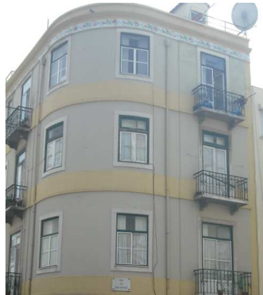
Figure 3.11 - Façade recently renovated
