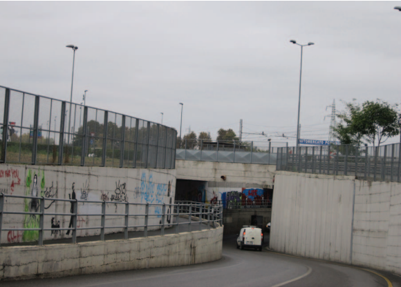
Photo I: Under pass to cross the road and railway.
