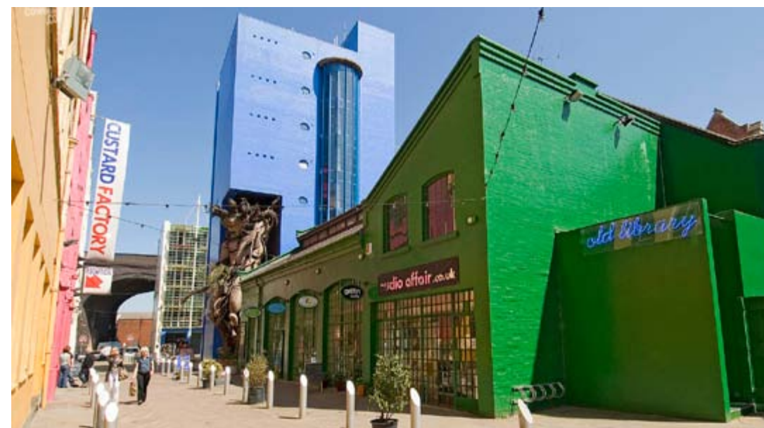
img035_CUSTARD FACTORY - Birmingham
