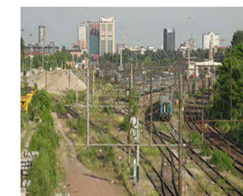
VIEW OF THE RAILWAYS TOWARDS PORTA NOUVA FROM FARINI BRIDGE
