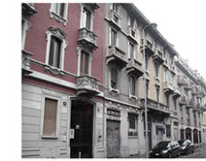
VIA APPRIKA, THE ABANDONED OFFICES AND LOFTS
