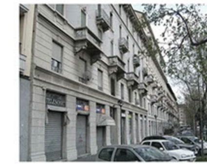
THE COMPACT AND DENSE FRONT LINE OF VIA VALTELLINA, TOWARD VIA FARINI
