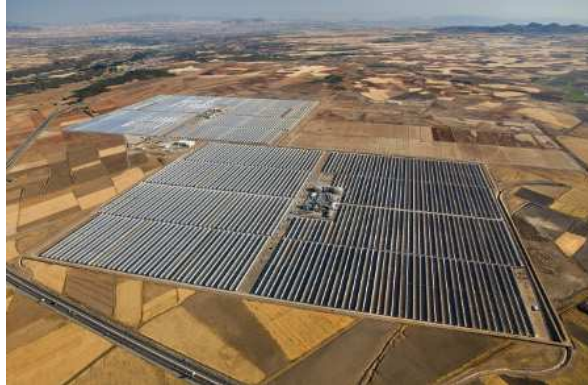
Figure 2-4: Andasol I and II. Power block and two-tank TES system surrounded by hectares of parabolic trough concentrators
