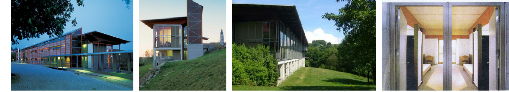
Guest Building for the Youth Education Centre Windberg, Niederbayern (prospetti ed interni)
