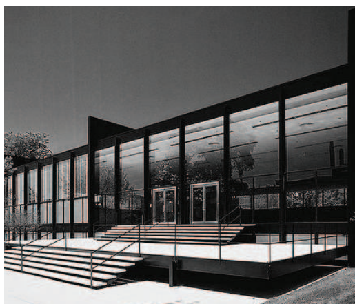
Fig. 5.2. - A sinistra: LUDWIG MIES VAN DER ROHE, Illinois Institute of Technology, Crown Hall , Chicago, Illinois, 1950 - 1956 (Foto storica).
