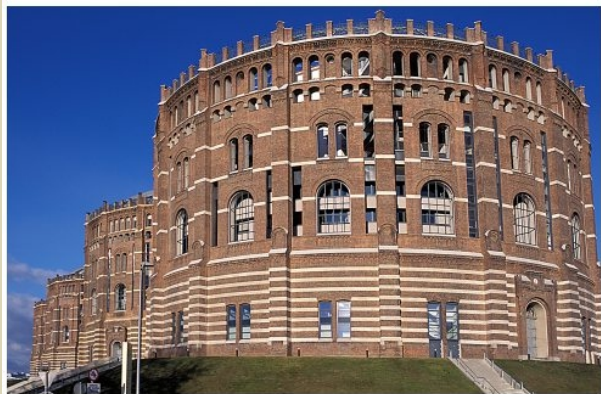
Fig 89 view of Gasometer after refurbishment
