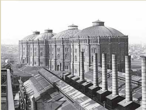
Fig 88 View of the Coal Plant
