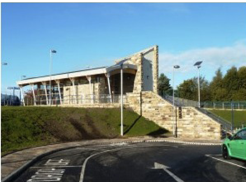
Fig. 4.1 Vista eterna, Accrington station, (Inghilterra)
