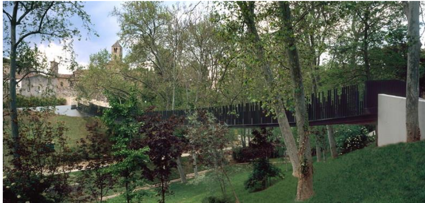
Vallparadís Footbridge by Pedelta Structural Engineers (2007)
