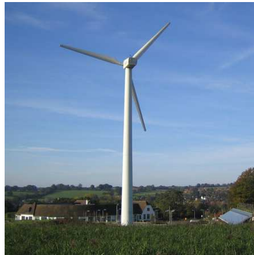
(b) Wind Turbine
