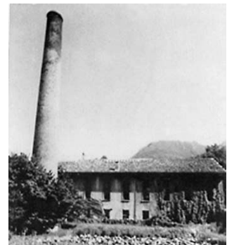
Figure 28 Chimney and west side of silk mill
