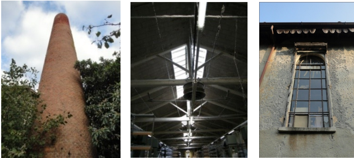
Figure 38 Building main features i.e., (Chimney, wooden truss and canopy)
