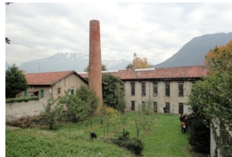
Figure 31 West view from the garden, Heating building – Chimney
