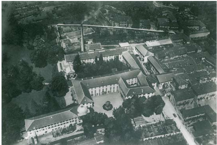
Figure 24 Aerial view of the Gavazzi complex in Valmadrera.
