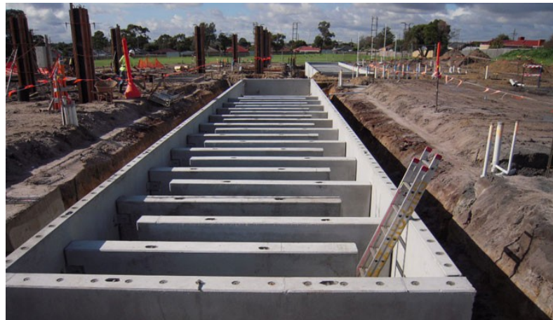
Figure 235 Thermal labyrinths concrete walls, taken from www.y2architecture.com.au
