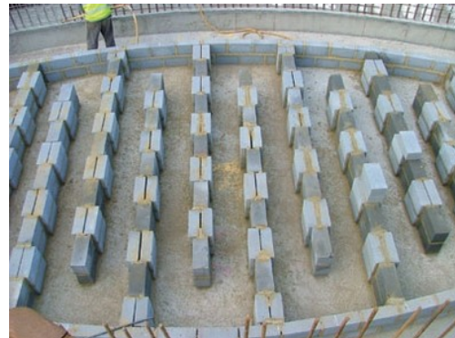
Figure 194 Labyrinths with Concrete blocks, taken from ( www.building.co.uk )
