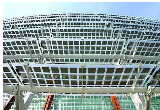
Figure 203 Glazed louvers with PV cells, extracted from ( www.colinfo.co.uk )
