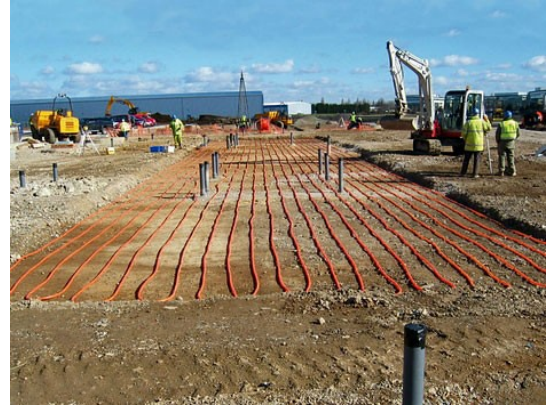
Figure 192 Pipe array being laid 3
