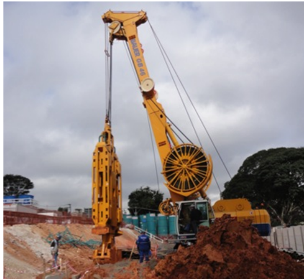
Figure 20: Hydraulic clamshell in Borba Gato station
