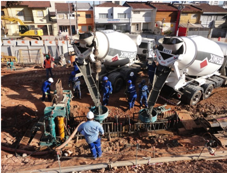
Figure 21: One of the concrete supplier's trucks
