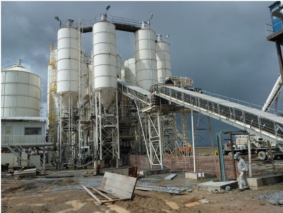
Figure 30: Concrete production in Belo Monte
