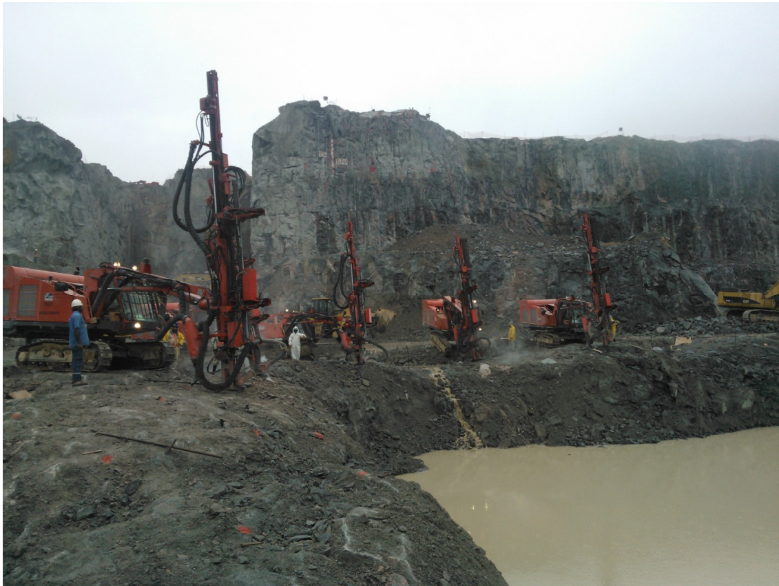
Figure 12: Rock excavation in Belo Monte
