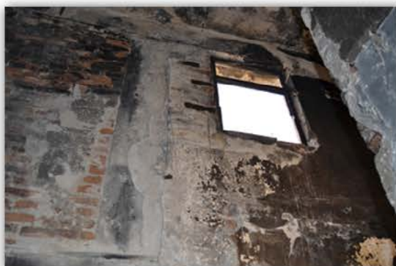
Picture 4.2.74 Room R20, D1 Wall
