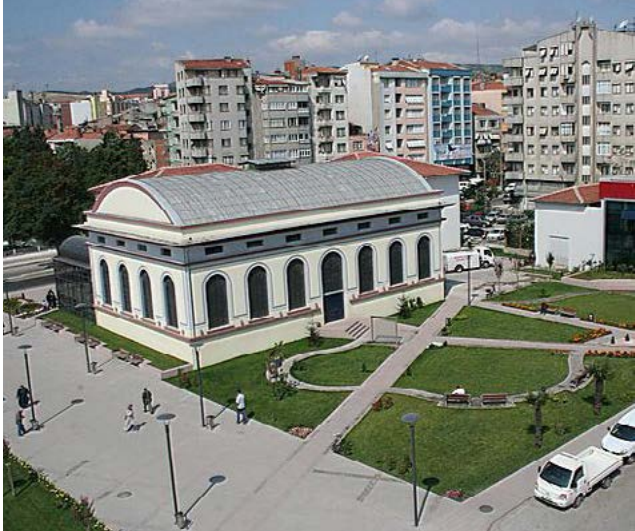
Picture 5.1.5 After restoration
