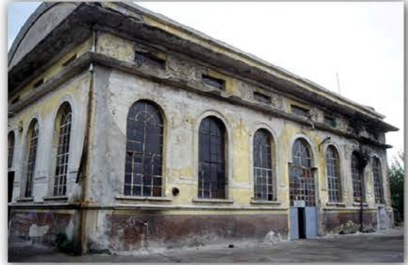
Picture 4.2.2 South-west facade
