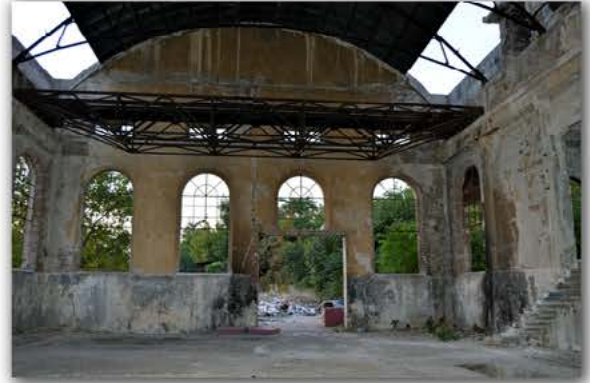
Picture 4.2.20 Room R01, D4 Wall
