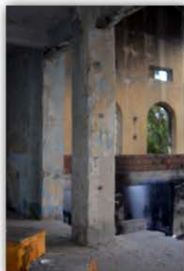
Picture 4.2.27 Room R07
