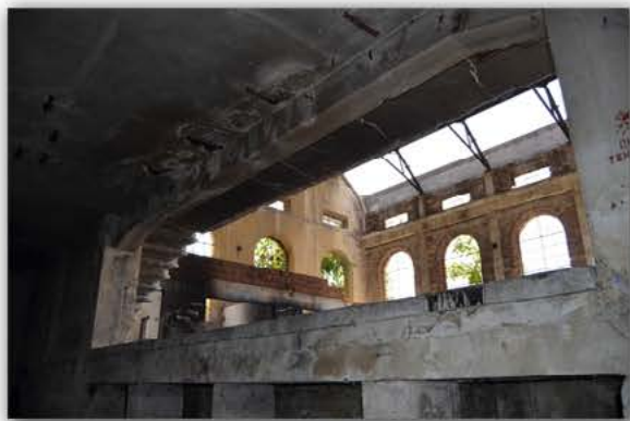
Picture 4.2.32 Room R09, D1 Wall
