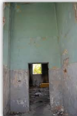
Picture 4.2.45 Room R11, D2 Wall
