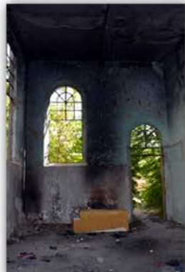
Picture 4.2.48 Room R12, D1 Wall
