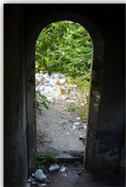
Picture 4.2.43 Room R10, Entrance
