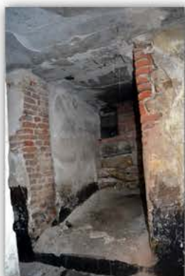
Picture 4.2.37 Room R09
