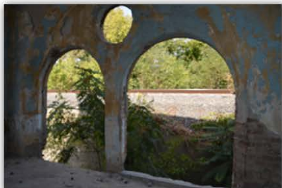
Picture 4.2.58 Room R14, D1 Wall
