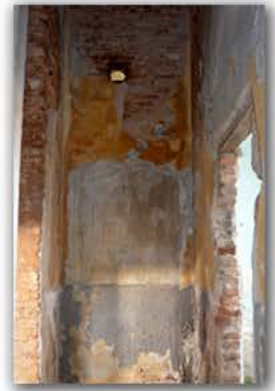
Picture 4.2.67 Room R17, D4 Wall
