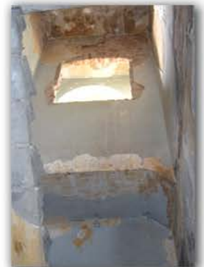
Picture 4.2.57 S05 Stair
