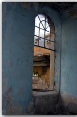
Picture 4.2.65 Room R16, D1 Wall
