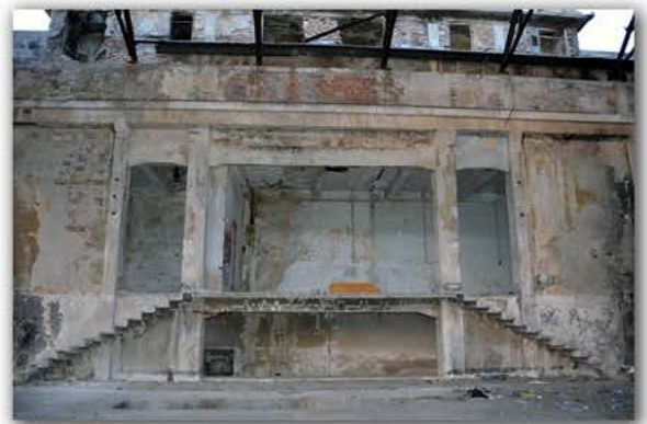
Picture 4.2.16 Room R01, D1 Wall
