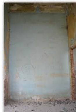
Picture 4.2.59 Room R14, D2 Wall
