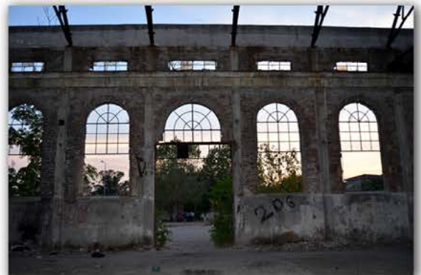
Picture 4.2.18 Room R01, D3 Wall
