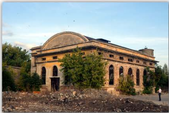
Picture 4.2.12 North-west facade
