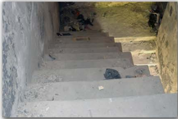
Picture 4.2.53 S05 Stair
