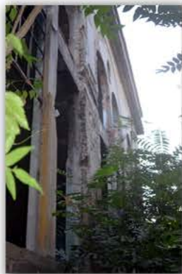
Picture 4.2.15 North-east facade
