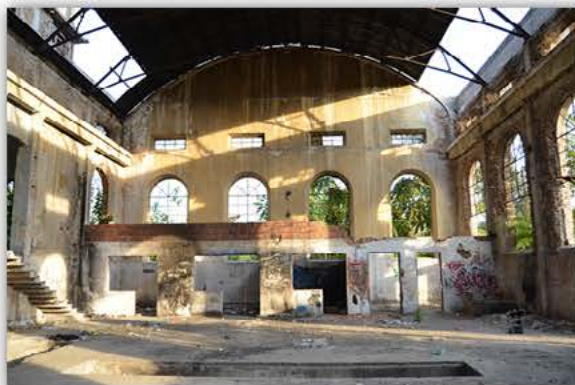
Picture 4.2.17 Room R01, D2 Wall
