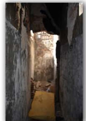
Picture 4.2.76 Room R20, D2 Wall
