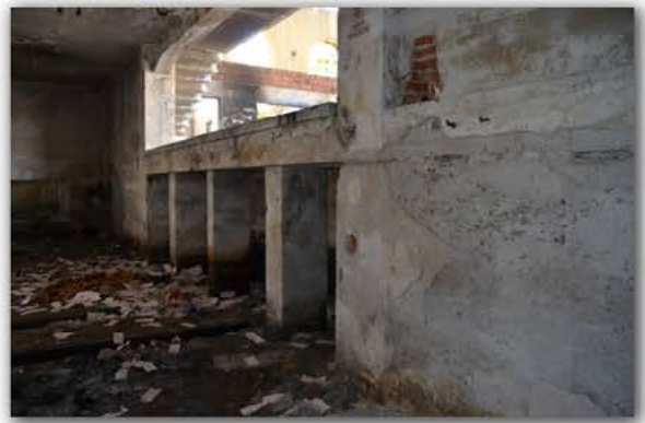
Picture 4.2.31 Room R09, D1 Wall
