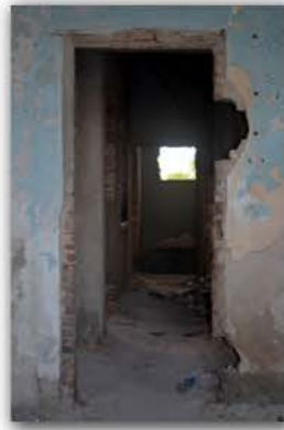
Picture 4.2.66 Room R16, D3 Wall
