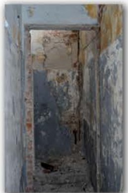
Picture 4.2.72 Room R19, D2 Wall
