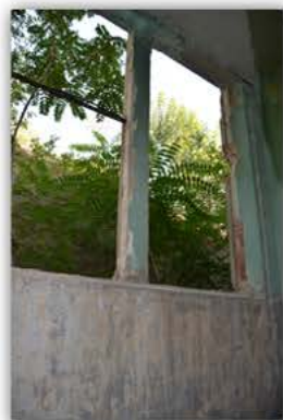
Picture 4.2.44 Room R11, D1 Wall
