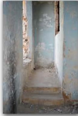
Picture 4.2.78 Room R21, D2 Wall
