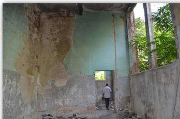
Picture 4.2.50 Room R12, D3 Wall
