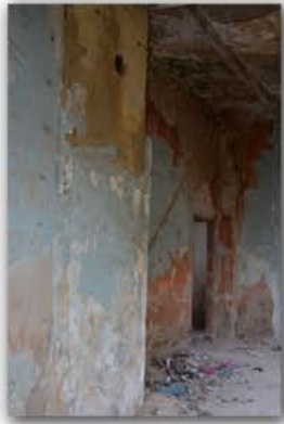
Picture 4.2.64 Room R15, D3 Wall
