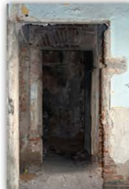
Picture 4.2.56 Room R13, D2 Wall
