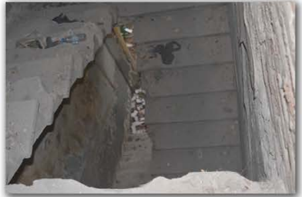
Picture 4.2.54 S05 Stair
