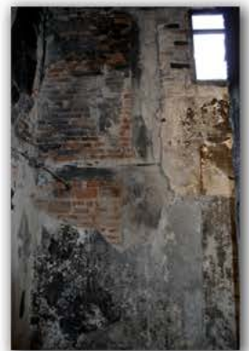
Picture 4.2.73 Room R20, D1 Wall
