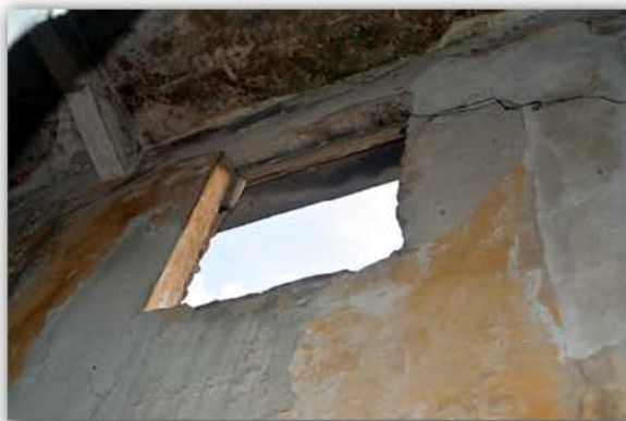
Picture 4.2.71 Room R19, D1 Wall
