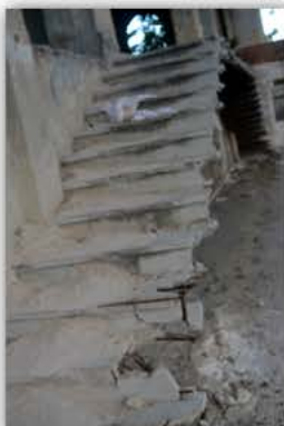
Picture 4.2.26 Room R01, S01 Stair
