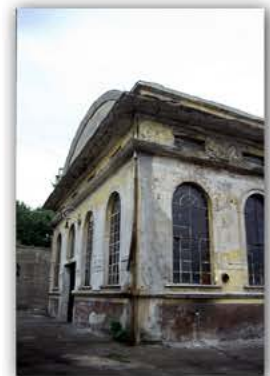
Picture 4.2.5 North-west facade
