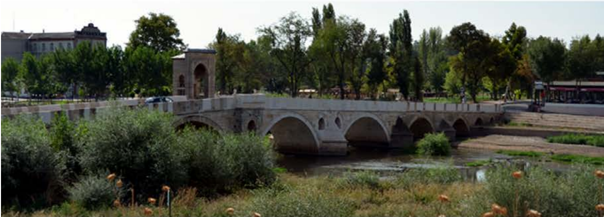
Picture 7 Ekmekçiöğlü Bridge
