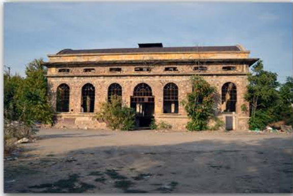
Picture 4.2.10 South-west facade
