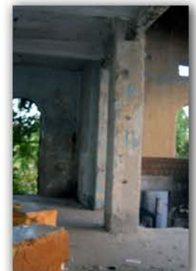
Picture 4.2.29 Room R07
