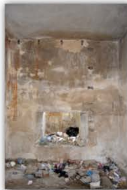
Picture 4.2.33 Room R09, D2 Wall
