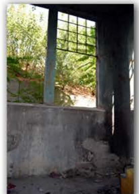
Picture 4.2.52 Room R12, D4 Wall
