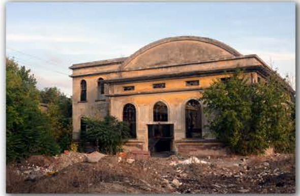
Picture 4.2.11 North-west facade
