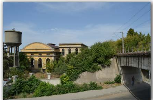
Picture 4.2.13 South-east facade
