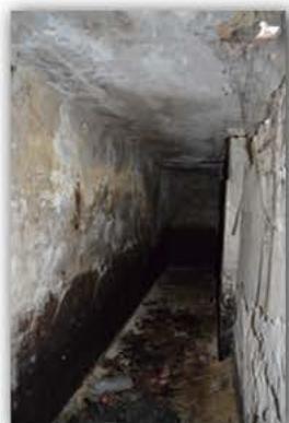
Picture 4.2.38 Room R09
