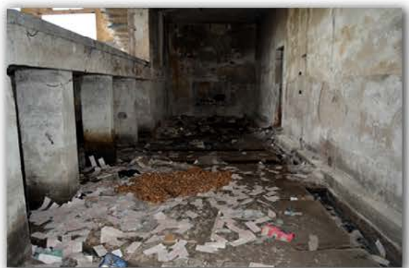
Picture 4.2.36 Room R09
