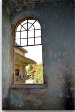
Picture 4.2.77 Room R21, D1 Wall
