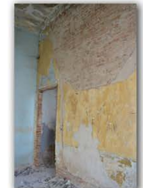
Picture 4.2.60 Room R14, D3 Wall
