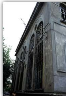
Picture 4.2.4 North-east facade
