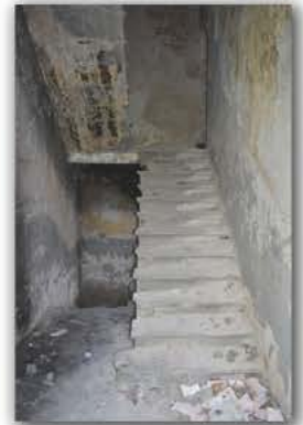
Picture 4.2.42 Room R10, S03 Stair
