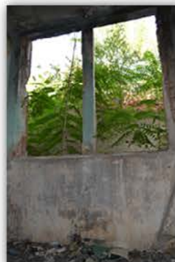
Picture 4.2.51 Room R12, D4 Wall
