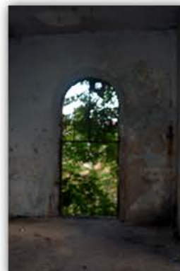
Picture 4.2.28 Room R06, D1 Wall
