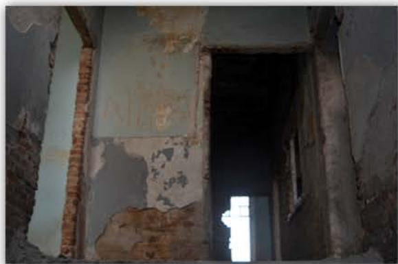
Picture 4.2.55 Room R13, D1 Wall
