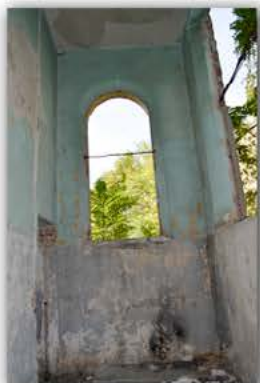
Picture 4.2.47 Room R11, D4 Wall
