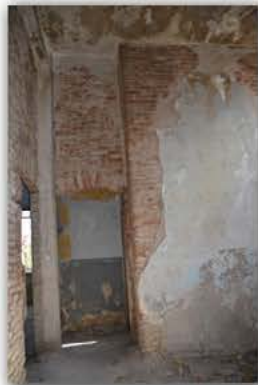
Picture 4.2.69 Room R17, D1 Wall
