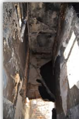
Picture 4.2.75 Room R20, D2 Wall
