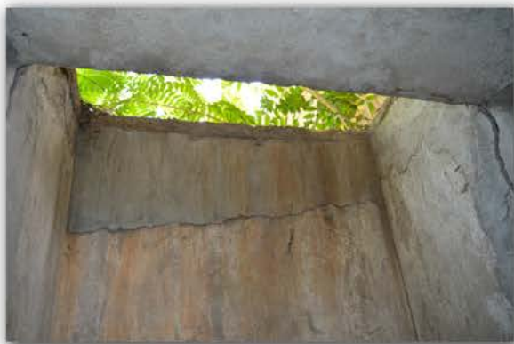
Picture 4.2.35 Room R09
