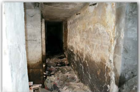
Picture 4.2.39 Room R09
