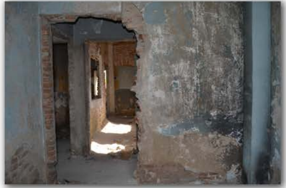
Picture 4.2.79 Room R21, D5 Wall
