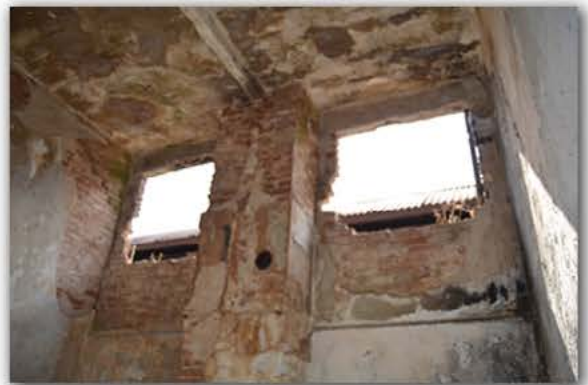
Picture 4.2.70 Room R17, D2 Wall
