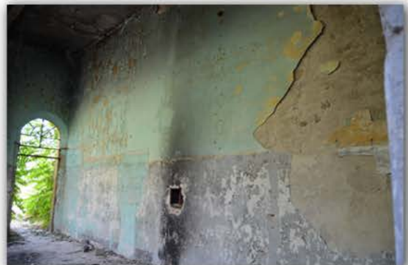
Picture 4.2.49 Room R12, D2 Wall
