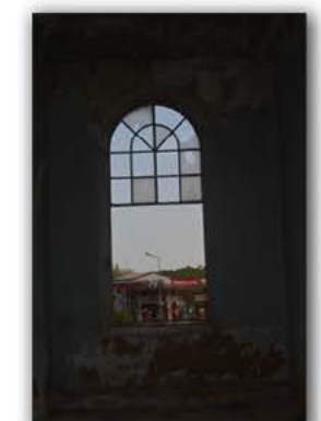
Picture 4.2.63 Room R15, D2 Wall
