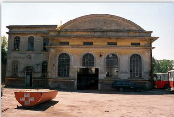
Picture 4.2.3 North-west facade
