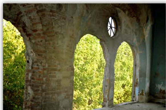
Picture 4.2.62 Room R15, D1 Wall
