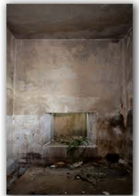
Picture 4.2.34 Room R09, D4 Wall
