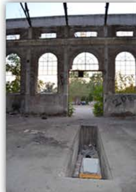
Picture 4.2.24 Room R01
