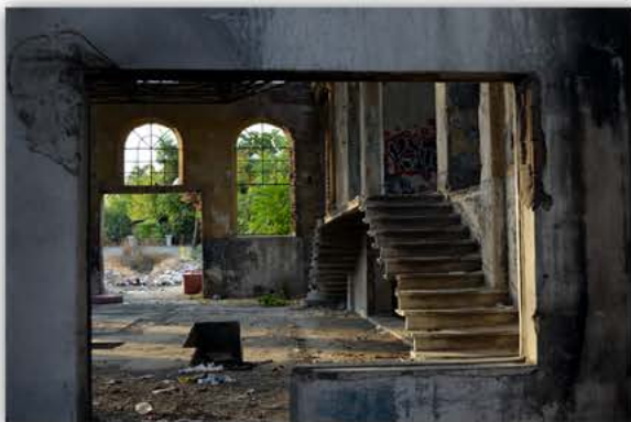
Picture 4.2.23 Room R02, D4 Wall
