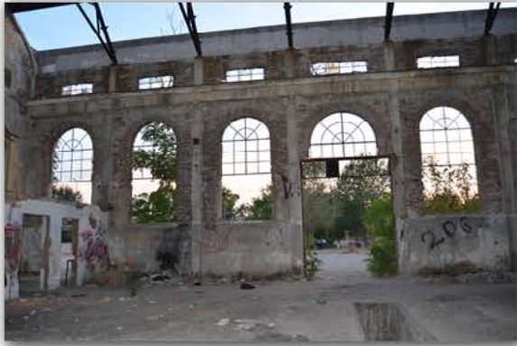
Picture 4.2.19 Room R01, D3 Wall
