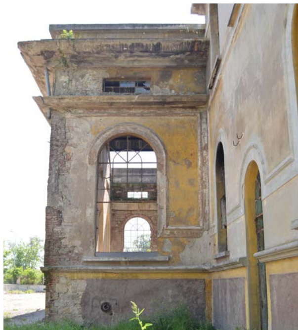
Picture 4.7 Water Out Pipe
