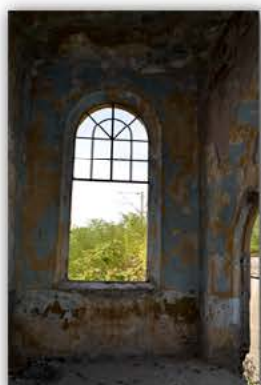
Picture 4.2.61 Room R14, D4 Wall
