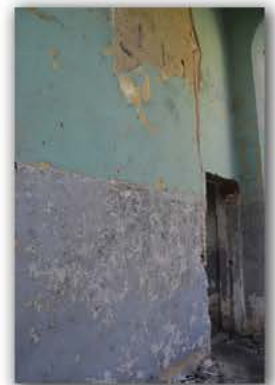
Picture 4.2.46 Room R11, D3 Wall
