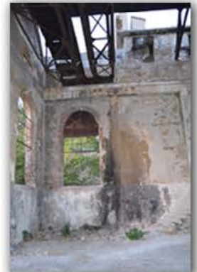
Picture 4.2.25 Room R01
