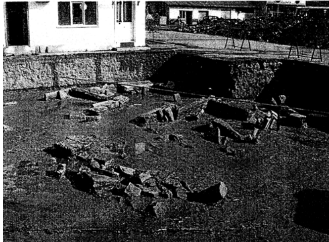
Picture 3.14 General view of the excavation
