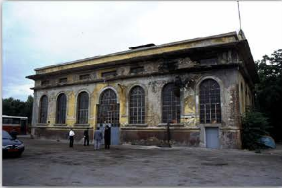
Picture 4.2.1 South-west facade
