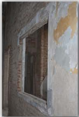
Picture 4.2.68 Room R17, D5 Wall
