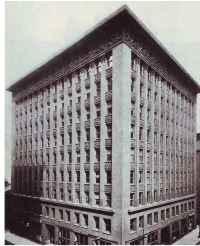
Sullivan e Adler, Wainwright Building | St Louis | 1891 32
