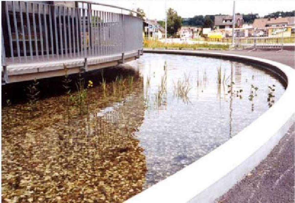
Figure 4.37 – Rainwater Storage Canal
