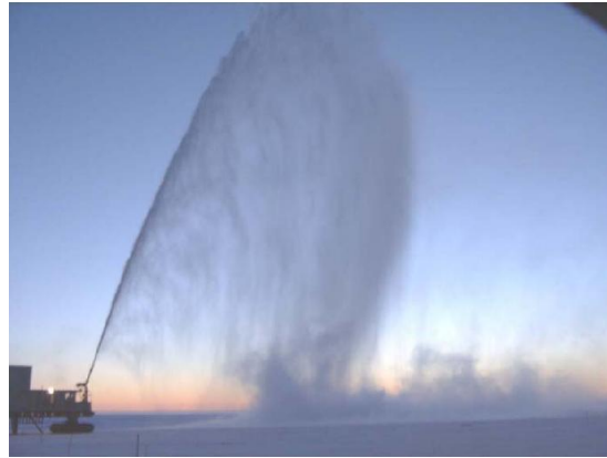
Figure 3.13- Ice island construction. Source: Blade
