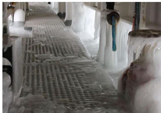
Figure 3.35- Frozen deck. Source: Termon
