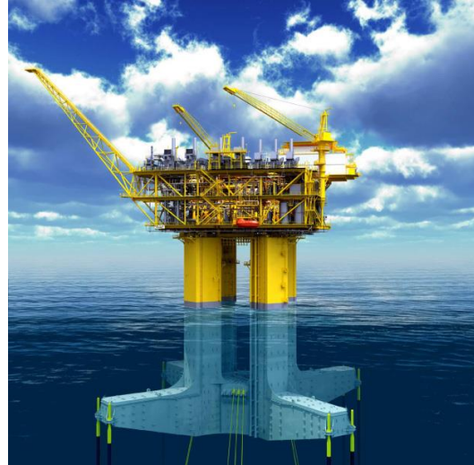
Figure 3.17- TLP. Source: modec.com
