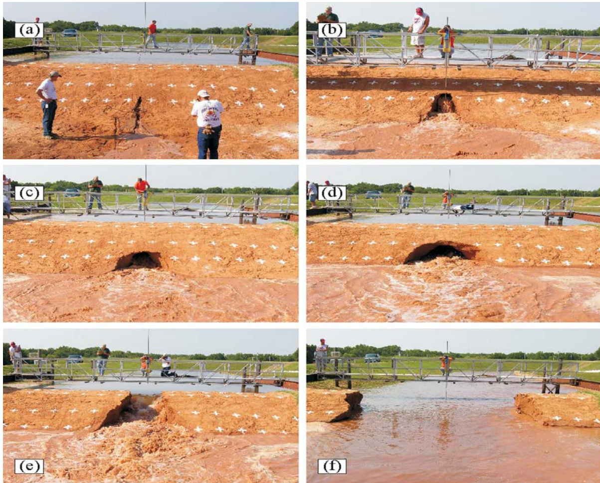
Fig. 6. 23: Dam breaching attributable to piping.
