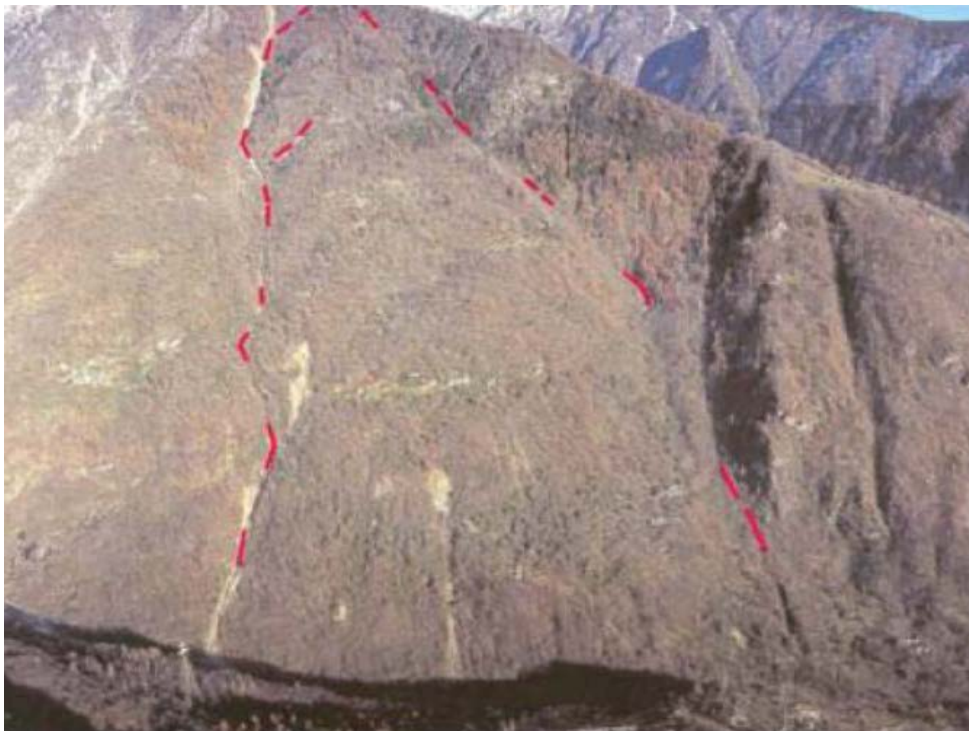
Fig. 4. 15: The body of Spriana landslide.
