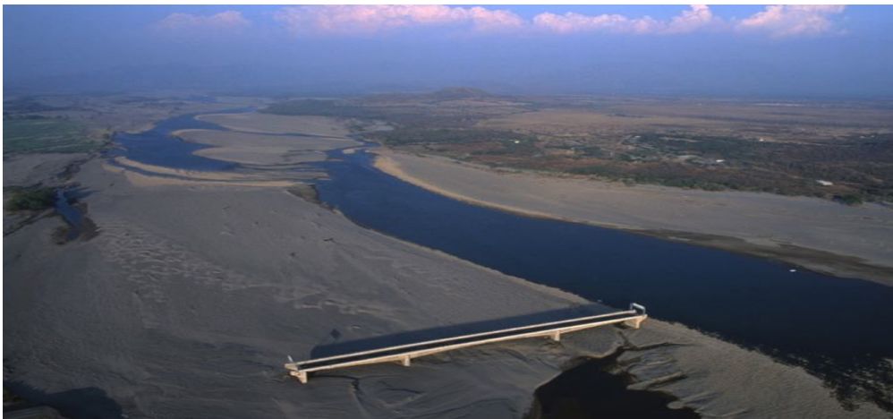
Fig. 1. 6: Choluteca Bridge, Honduras after Hurricane Mitch. 1998.
