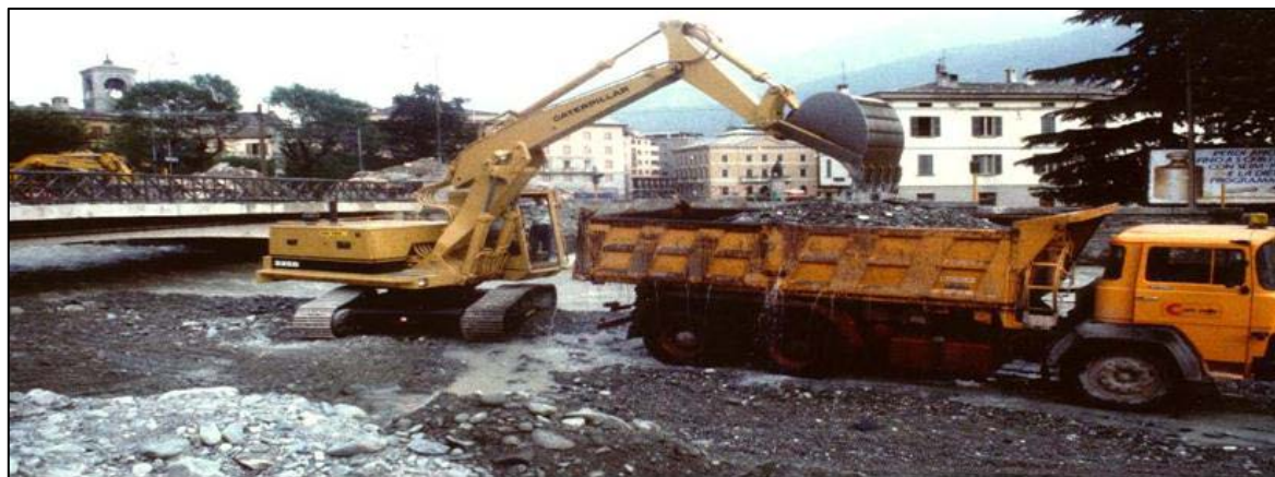
Fig. 4. 11: Dredging operations after 1987 flood.
