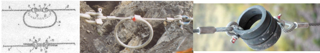
Figure 1-9 Types of absorption elements in rock fall protection meshes: hidden length with friction between ropes (left), bent steel pipe circle narrowing under tension (center) and elongating spiral spring (right) (taken from [17]).
