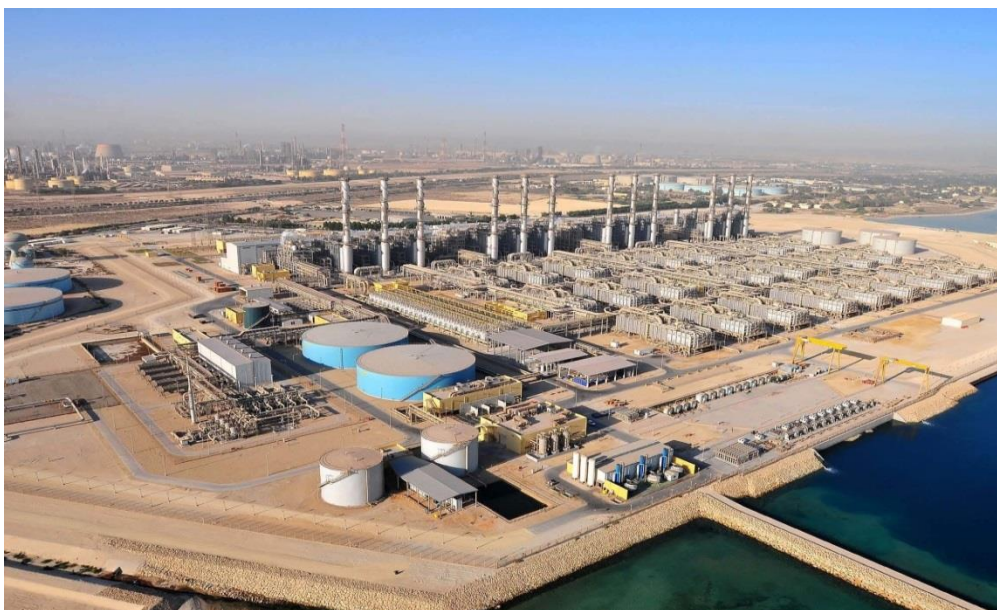
FIGURE 6. THE MARAFIQ PLANT IN SAUDI ARABIA. IN THE PICTURE, CLOSER TO THE SEA IT IS POSSIBLE TO SEE ALL THE 27 MODULES THAT FORM THE DESALINATION PLANT, AND BEYOND THEM, THE POWER PLANT.
