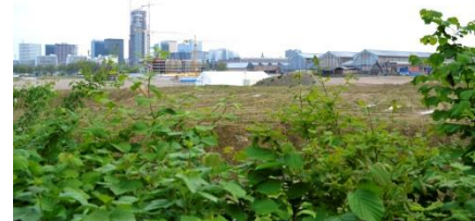
View from the garden towards the construction site
