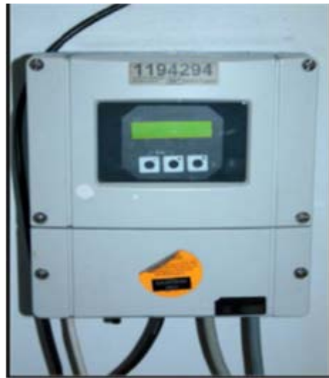
Figure 2.2: Flow meter.
