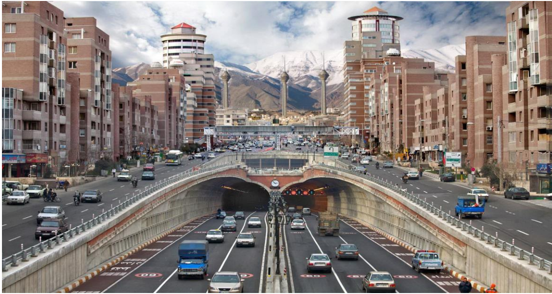
Figure 1: Tehran Tohid Tunnel
