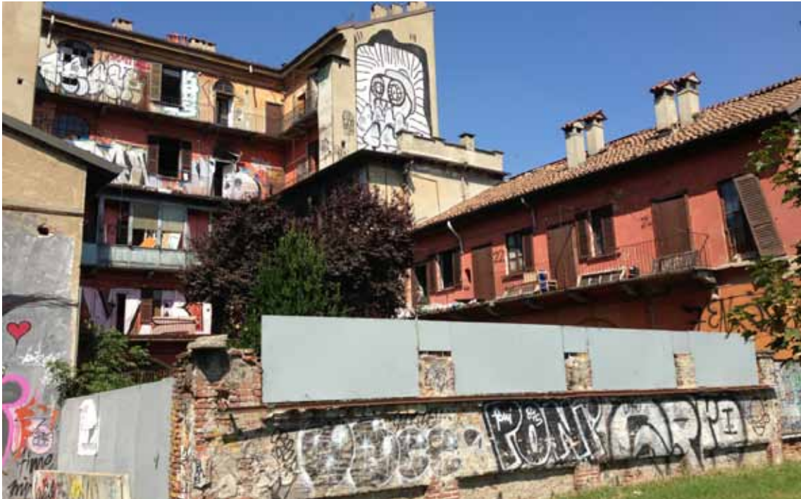
10 - Abandoned building in Ripa di Porta Ticinese
