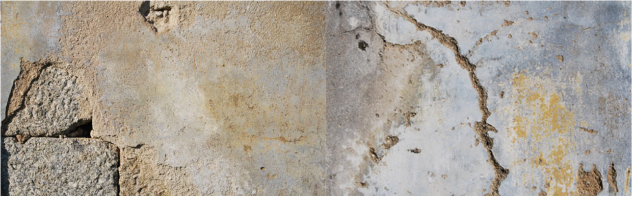
Figure 26: Detailed views from the Binding Mortar and Plaster on the Walls.
