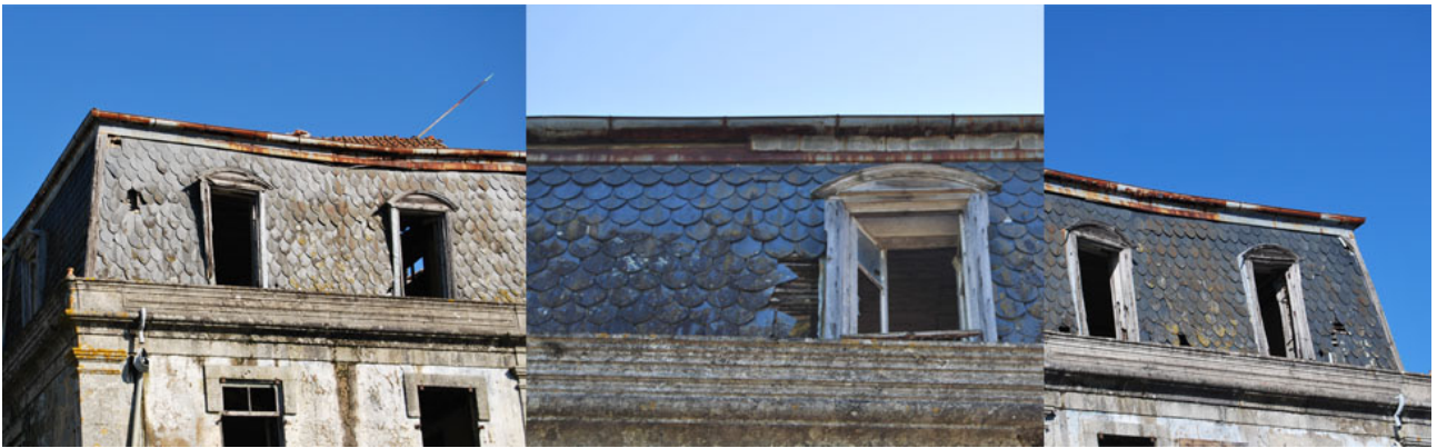
Figure 28: Views from the Tiles used on the Mansard.
