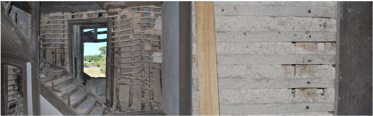
Figure 19: View of the Tabique Interior Wall. Detail of the Wall Composition.
