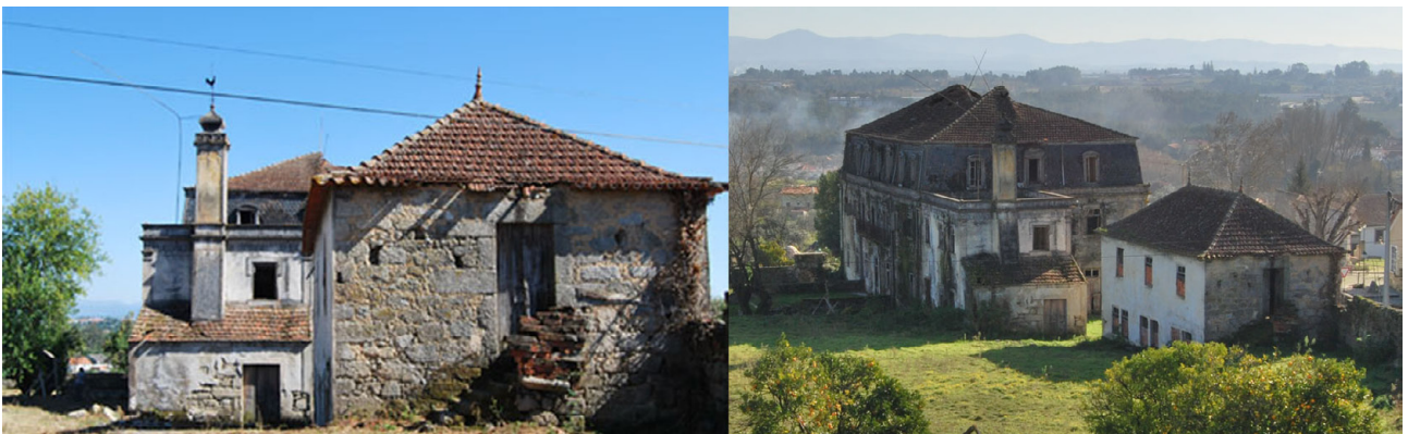
Figure 29: View of the tiles on the roofs.
