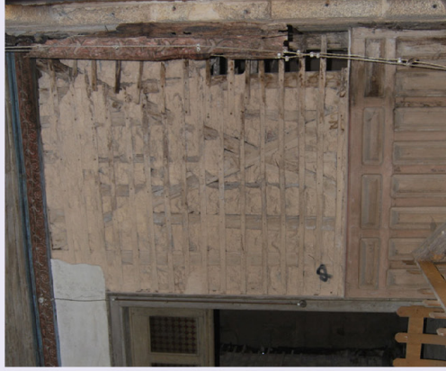
View from a "Frontal" Wall on the Ground Floor.
