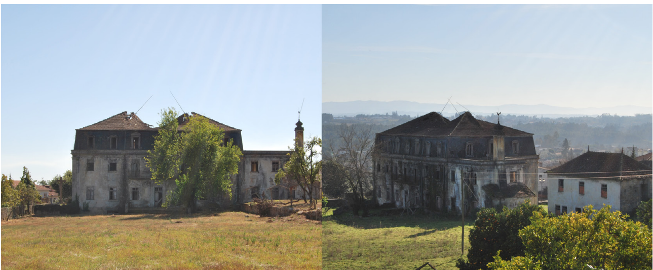
Figure 63: Views from the whole in the centre of the roof.
