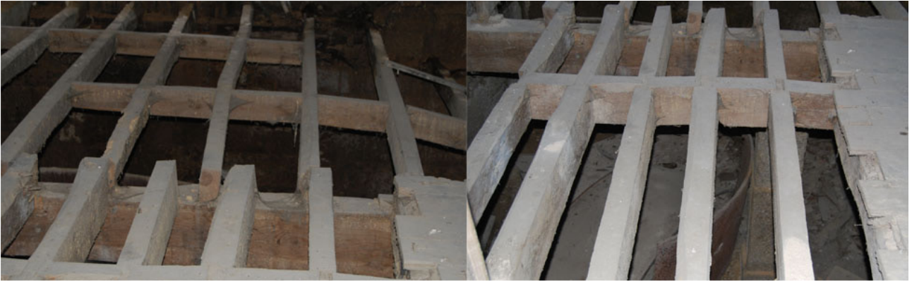
Figure 21: Detailed Pictures of the Wood Structure of the Floors
