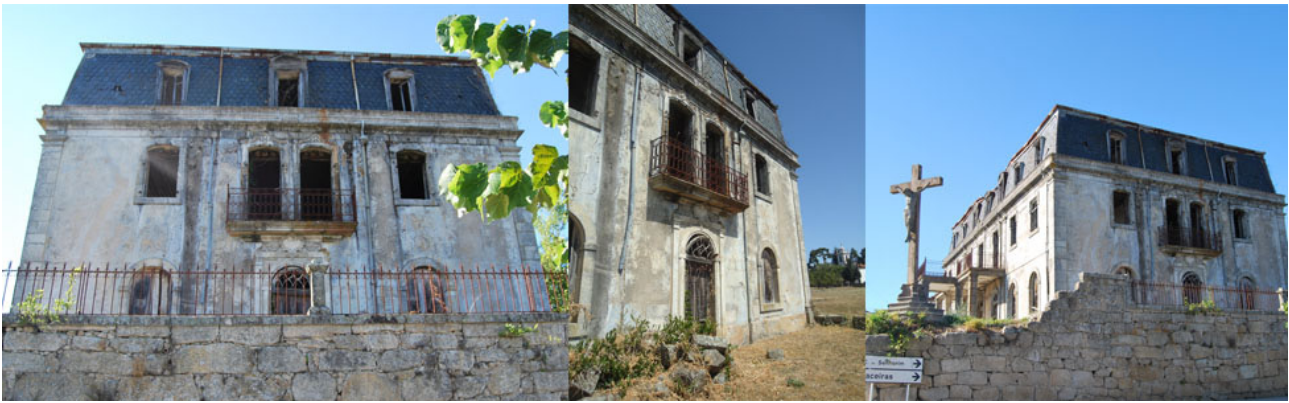
Figure 38: View from the South-East Façade. Closer view of the balcony. View from the opposite side Avenida Aristides de Sousa Mendes
