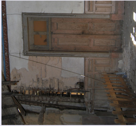
View of the "Frontais" Wall with the different Plaster layers.
