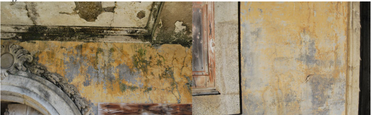
Figure 27: Detailed views from the remains of the ocre paint under the main façade's balcony.
