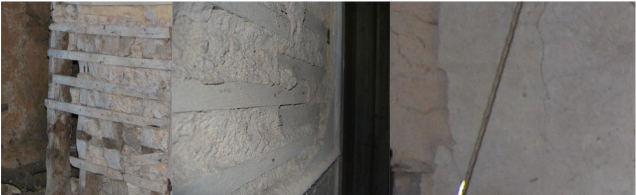
Figure 20: First, Second and Third Layers of the Wall's Filling Respectively.
