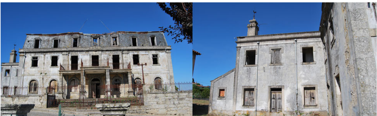
Figure 36: View of the South-West Façade. View of the Services building.
