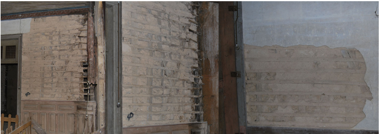
Figure 18: View from the Frontal Walls on R01 and R14
