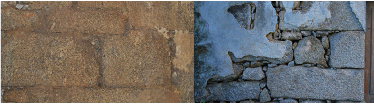
Figure 24: Detailed Pictures of the Granite Walls
