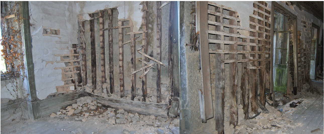
Figure 65: View from the Interior Bearing Walls on the First Floor.
