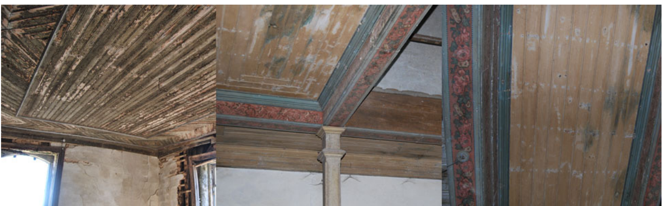
Figure 42: View from the 2° Floor Ceiling and details of the Hall’s Ceiling.
