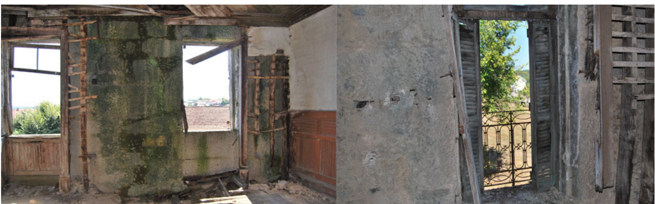
Figure 17: Interior views of the Granite Bearing Walls
