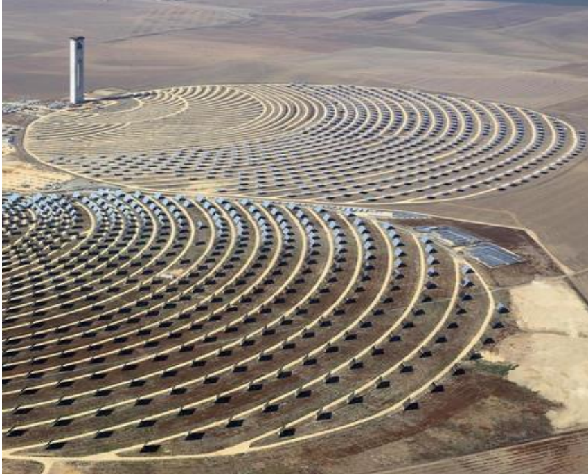
Figure 3-8 Heliostat field of PS10 and PS20 in Seville, Spain
