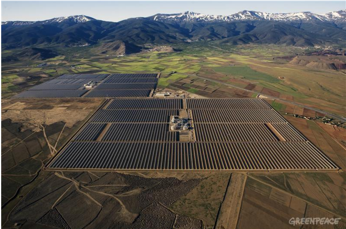
Figure 3-2 Andasol I and II parabolic trough power plants
