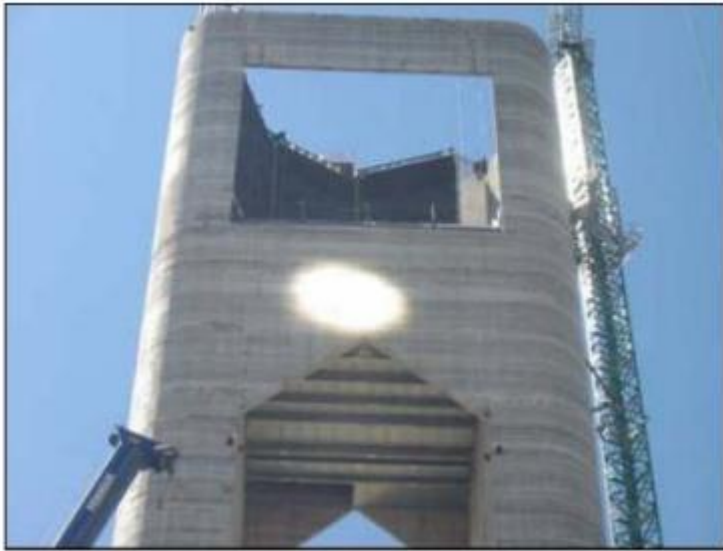
Figure 5-16 the cavity receiver of PS10 plant under construction
