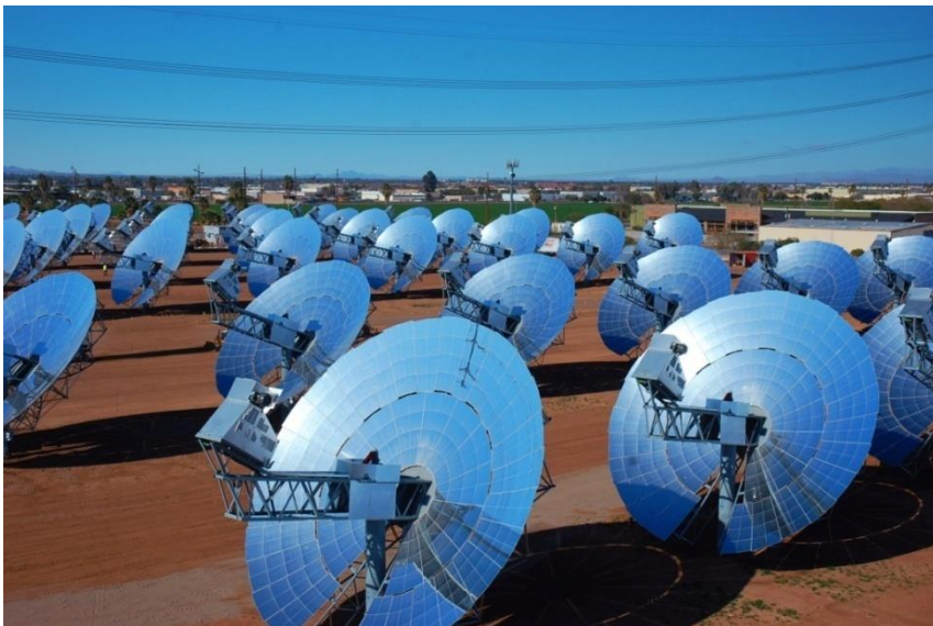
Figure 3-5 Parabolic dish field
