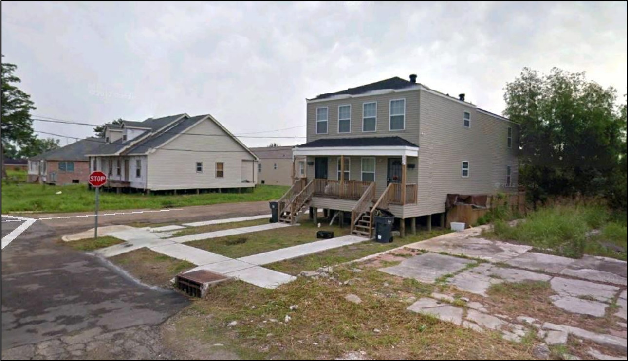
Figura 24 - Case ricostruite con piano rialzato in Gordon Street a Lower Ninth Ward, New Orleans.
