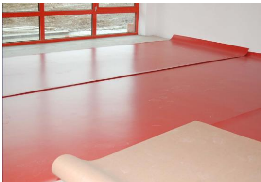
Fig. 225 Posa in opera linoleum
