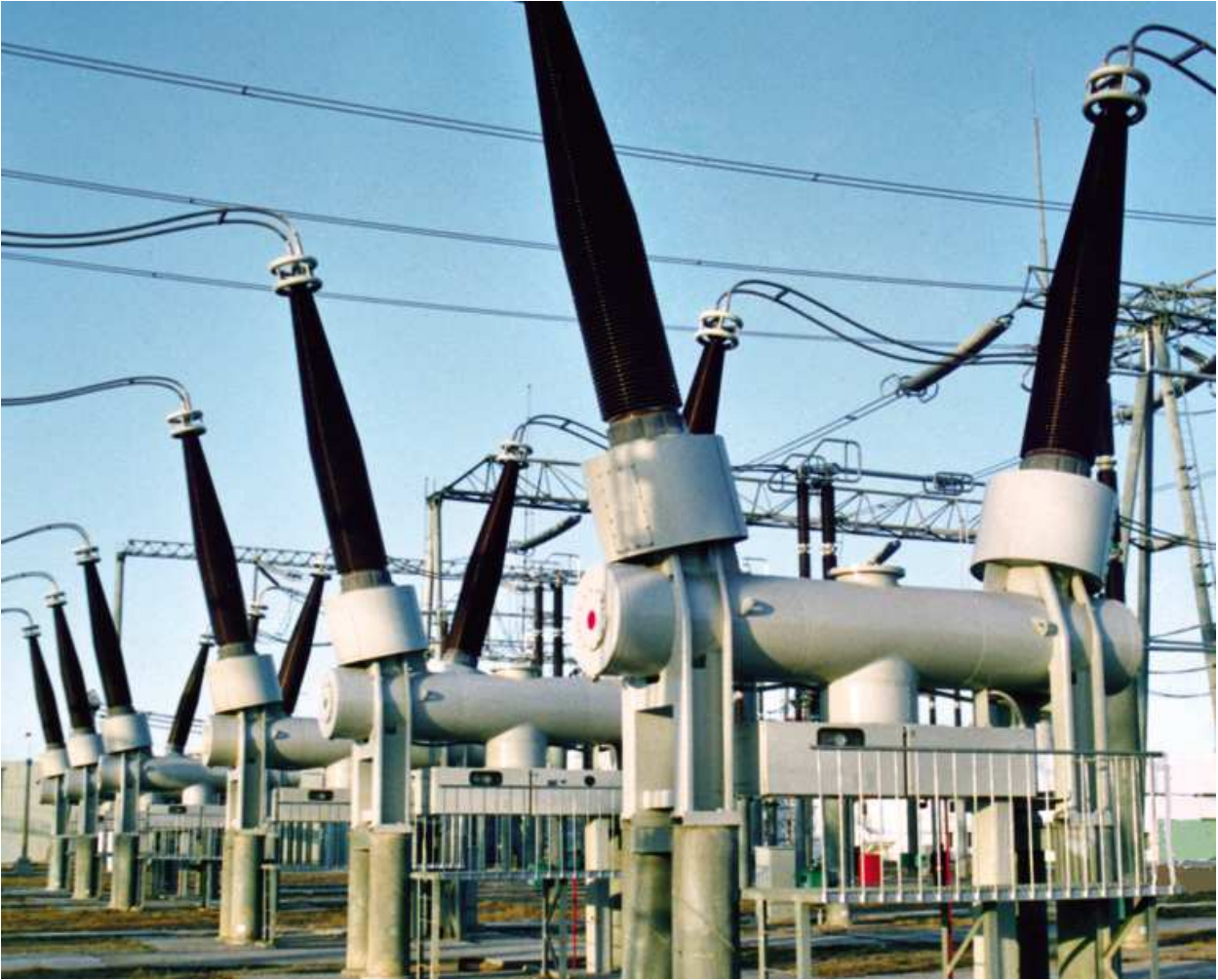
Figure 2.2 - 420 kV GIS circuit-breaker, equipped with bushings for the connection to the line, commonly named “dead tank circuit-breaker”, because the enclosure that contains the breaking mechanism is grounded.
