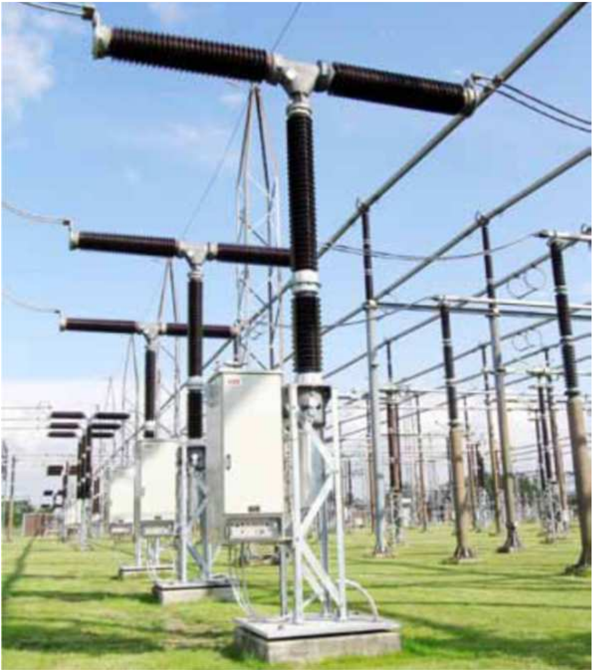
Figure 2.1 - AIS circuit-breaker, commonly named “live tank circuit-breaker”, because the enclosure that contains the breaking mechanism is at high voltage.
