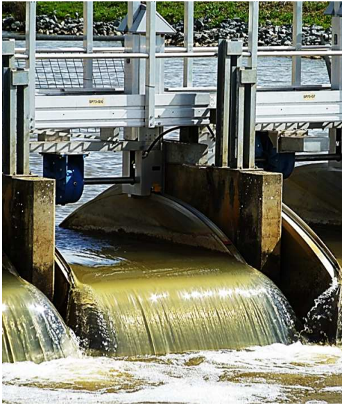
(a) Automated over-shot gate in a main channel
