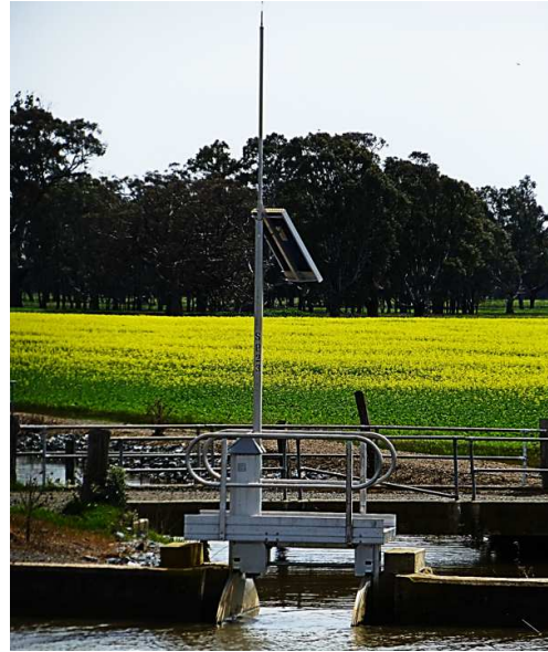
(b) Automated over-shot gate at off-take point
