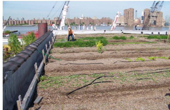
fig2.58 irrigation system and planting beds.
