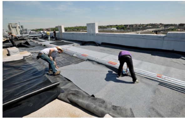
fig2.57 installation of waterproofing membrane and plumbing system
