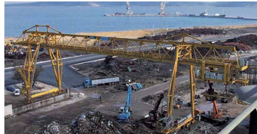
Figure 2.1. line of cranes working at the scrapyard Source : http://www.danieli.com
