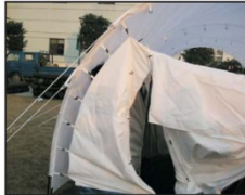
Pull up the inner inserting the toggles in the relative eyelets
