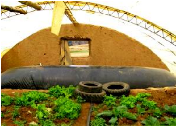
Figura 4.56 Dome - roof digester.
