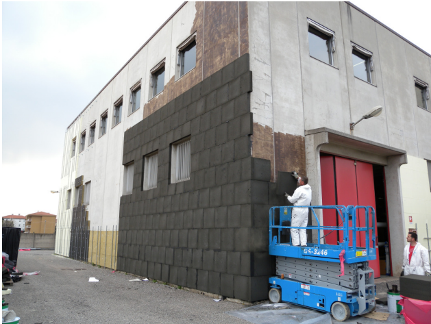
Figura 3.28 Posa in opera isolante Foamglas
