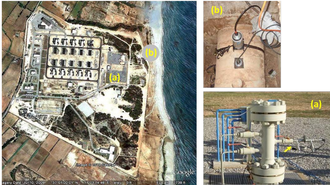
Figure 6.5. Satellite view: TMPC TRANSMED station of Cap Bon (Tunisia) and sensor location.
