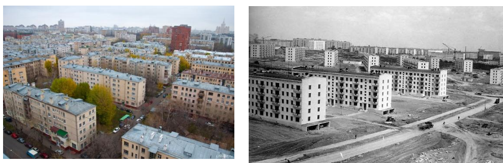
Figure 2.7 Soviet mass-housing construction
