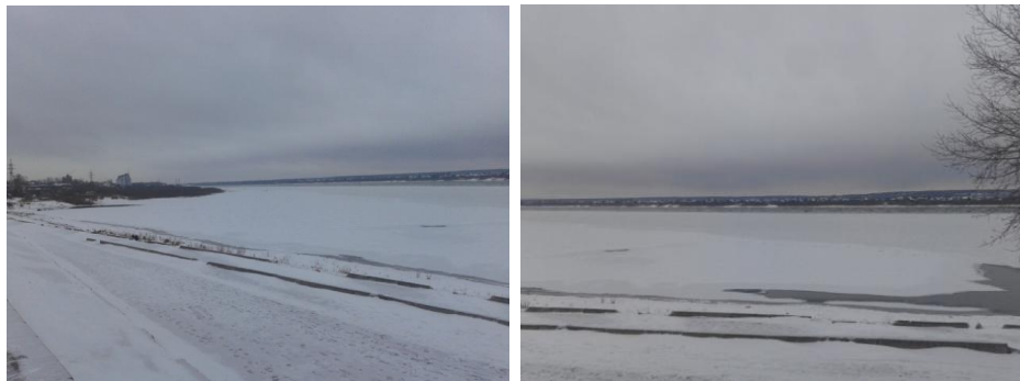
Figure 6. 9 The current view of the embankment
