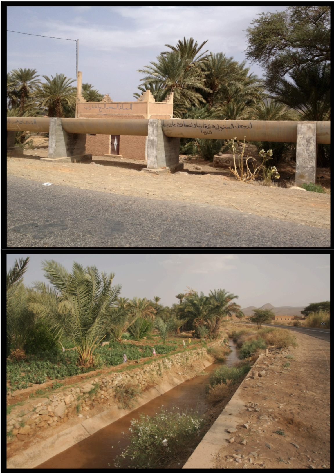
Figure 24: Irrigation system in the Draa Valley (source : Author)
