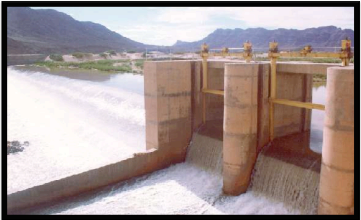
Figure 25: the Mansour Ad-Dhabi dam
