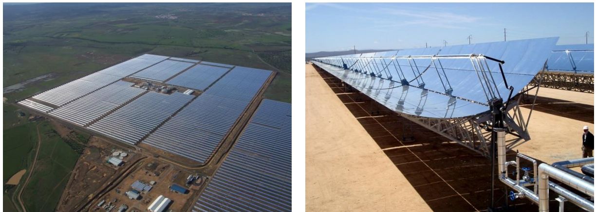
Figure 1.8 Aerial view of the Extresol 2 plant (left) and picture of a parabolic trough assembly
