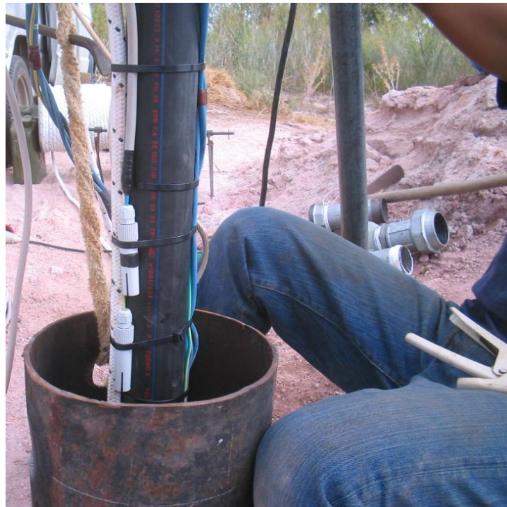
Figure 3.17 Standard tie mechanism used in the underwater pumping systems and clamping tool
