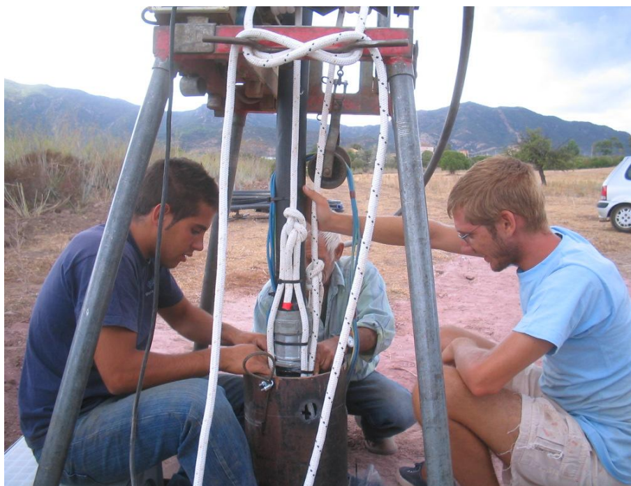
Figure 3.5 Winch to drop the underwater pumping system into the well
