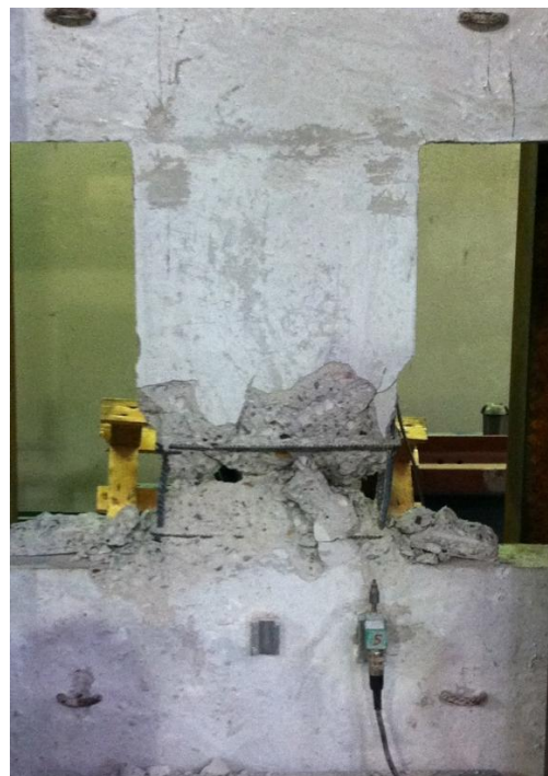
Figure 6.13 – Coupling beams with complete reinforcement at final step of displacement
