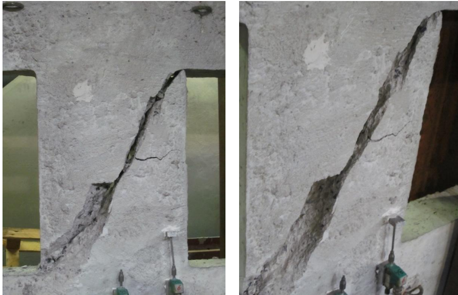
Figure 6.2 – Diagonal cracking of the beam without any reinforcement
