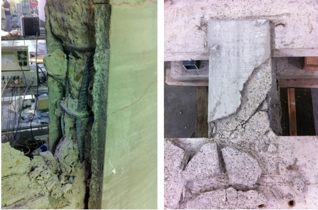
Figure 6.32 – Coupling beam retrofitted with HPFRCC at 2% pre-damage level – Failure of the beam
