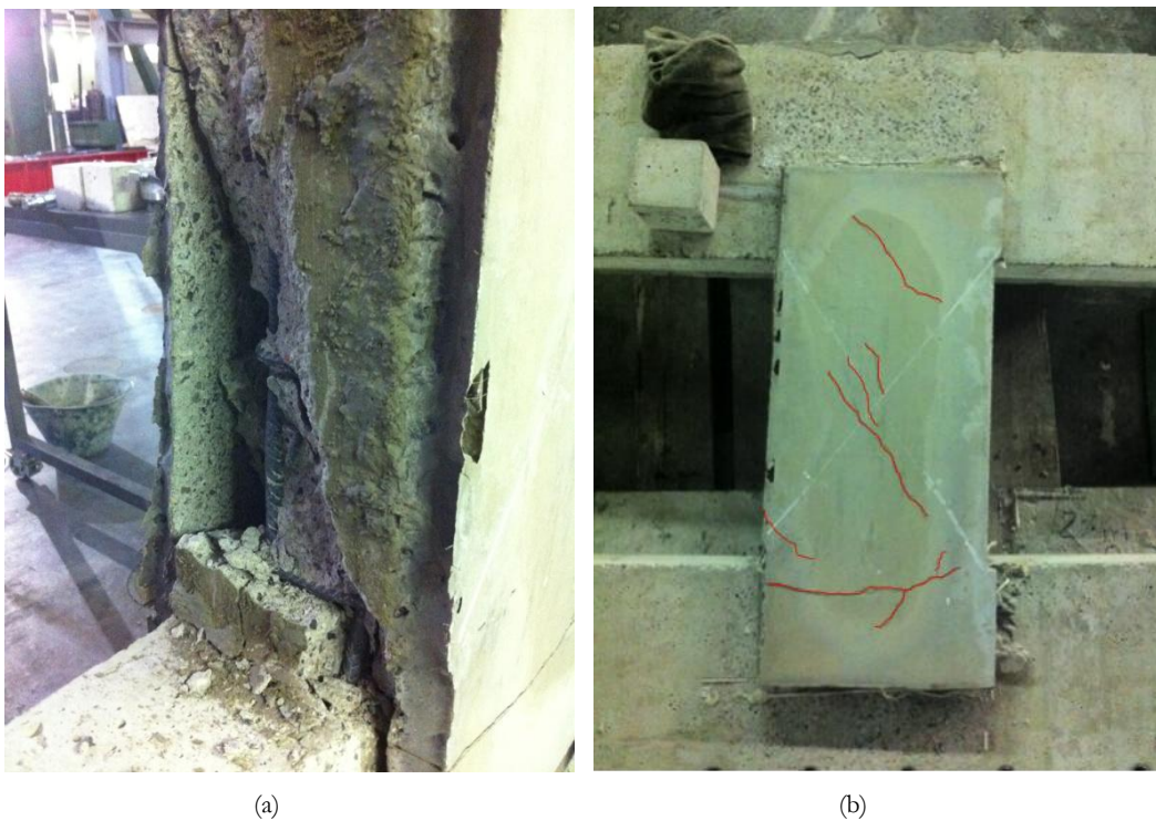
Figure 6.27 – Coupling beam retrofitted with HPFRCC at 1% pre-damage level monotonic: (a) crushing failure and (b) visible distributed cracks
