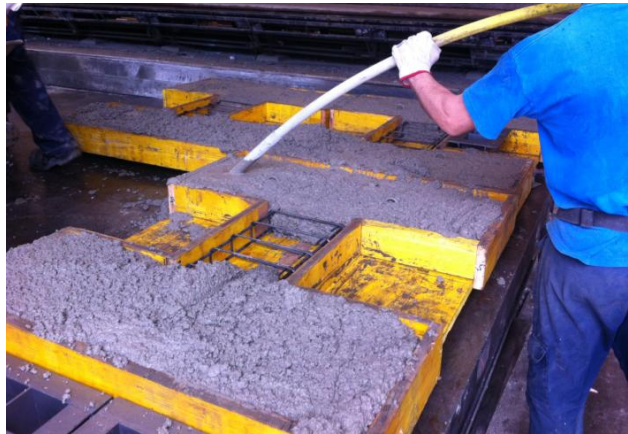
Figure 5.19 – Pouring and vibration of concrete
