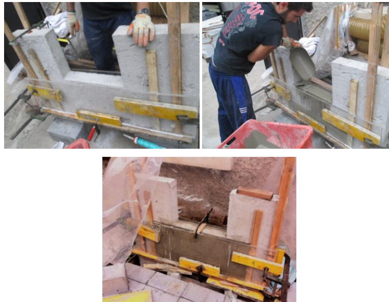
Figure 5.21 – Casting process of HPFRCC
