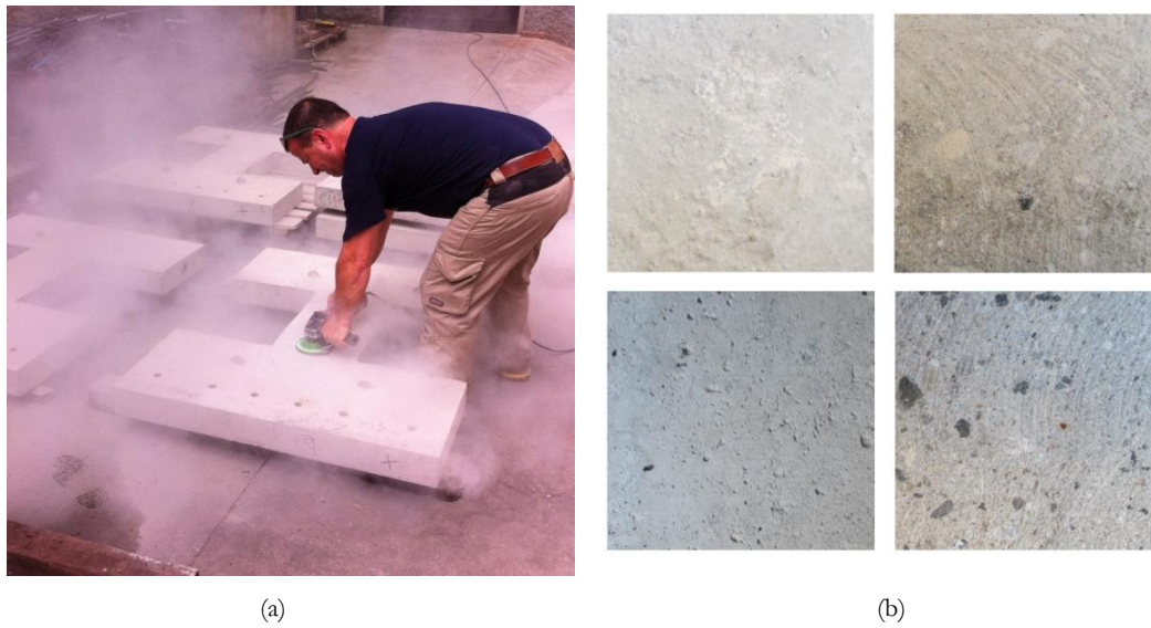
Figure 5.20 – (a) Roughening technique and (b) before and after treatment: top-upper surface; bottom-lower surface
