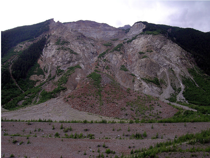
Figure 2.29: Landslide of Val Pola (Valtellina area, in Sondrio province), came off the 28 th July 1987.
