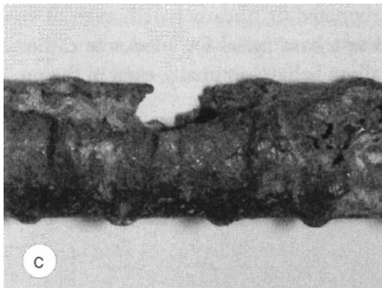
(c) Pitting corrosion.
