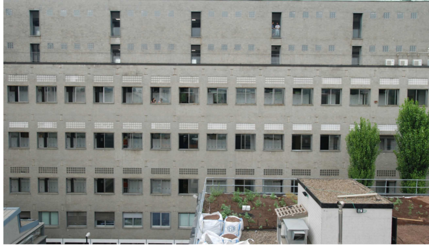
Fig. 5.21. ‘Nave building’ dataset: a pictures of the analysed building, due to the presence of a large tree in front of the façade a large occluded area has resulted in the final point cloud .
